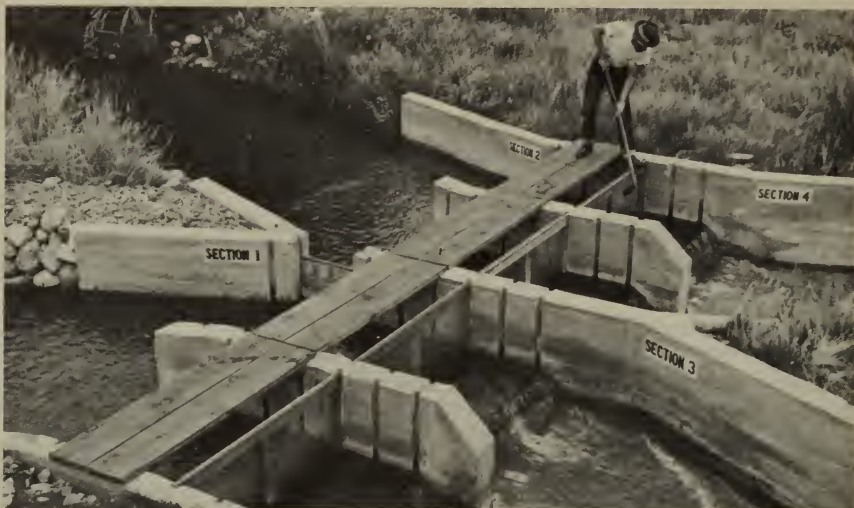
Convict Creek, Calif., experimental stream area showing middle-water control and screen structure. The four sections may be individually dewatered for population and survival counts.
