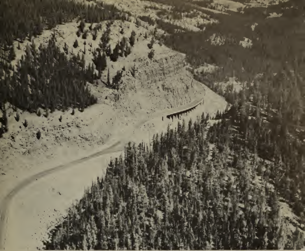
Rockslides caused by earthquakes in Yellowstone National Park in August, 1959, required extensive repairs to roads and buildings, amounting to several million dollars.
