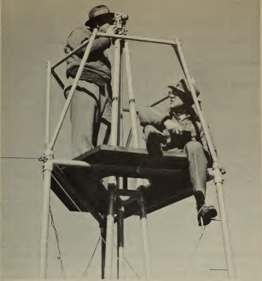
Survey topographic engineers measuring angles with a theodolite atop portable tower.
