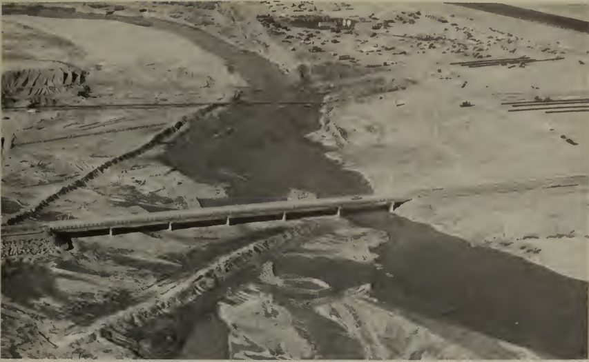
Four Corners Oil Field. Bridge built by Bureau of Indian Affairs across San Juan River helps in development of resources on Navajo Indian Reservation.
