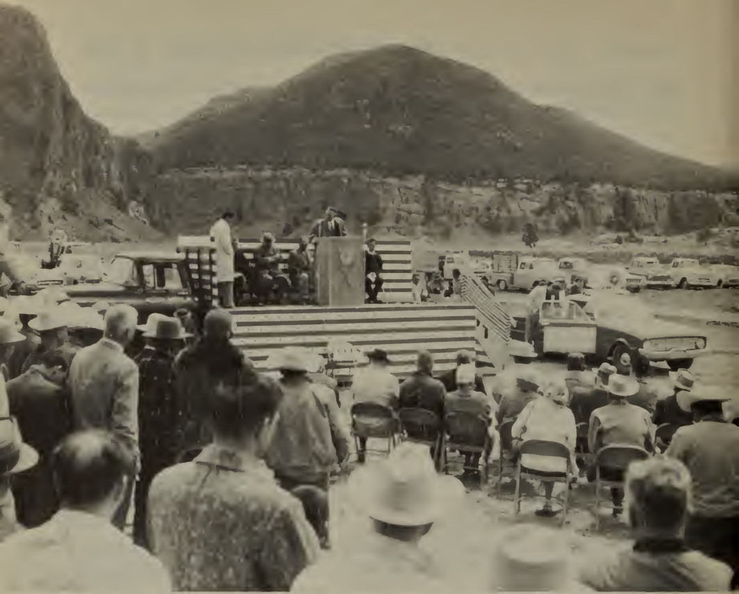
Ground-breaking ceremonies for the new tribal sawmill on the Navajo Reservation in New Mexico. Recent inventories of the Navajo timber resources showed that the annual cut could be substantially increased under a sustained yield management program.
