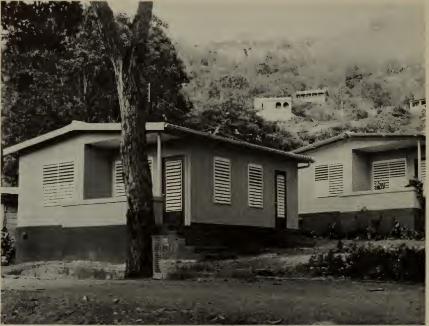
A single family unit of the Virgin Islands Emergency Housing Program.
