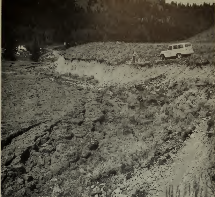
This is Red Canyon fault east of Blarneystone Ranch, a freshly made fault scarp caused by the Hebgen Lake, Mont., earthquake.
