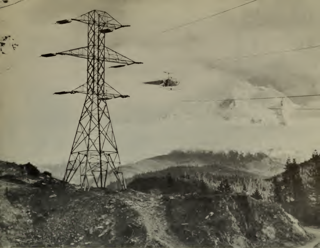
A Bonneville Power Administration helicopter patrols one of the double circuit steel transmission lines, bringing power down the Columbia gorge from the Mid-Columbia plants of the U.S. Columbia River Power System.
