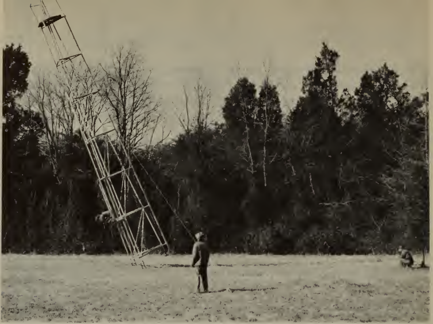
Erecting portable observing tower for triangulation mapping observations.
