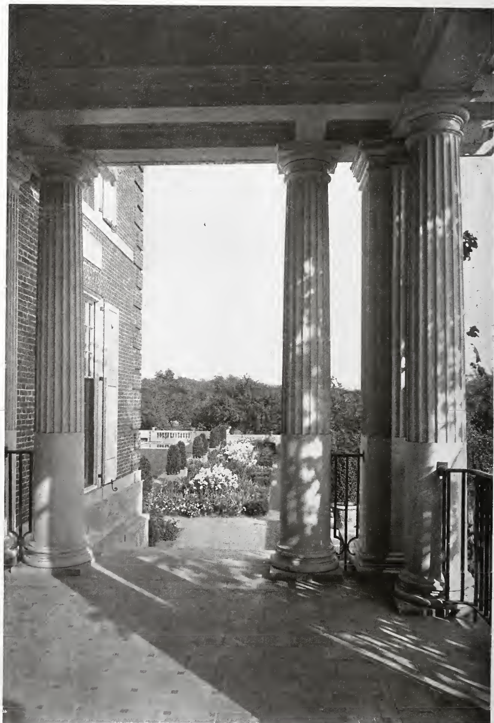
DETAIL—RESIDENCE OF GEO. L. NICHOLS. ESQ. Katonah, N. Y. Chas. A. Platt, Architect.
