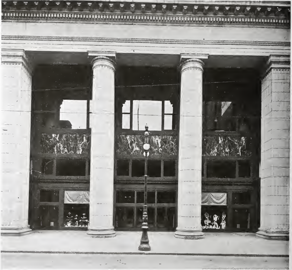
ENTRANCE DETAIL—THE WANAMAKER BUILDING.
