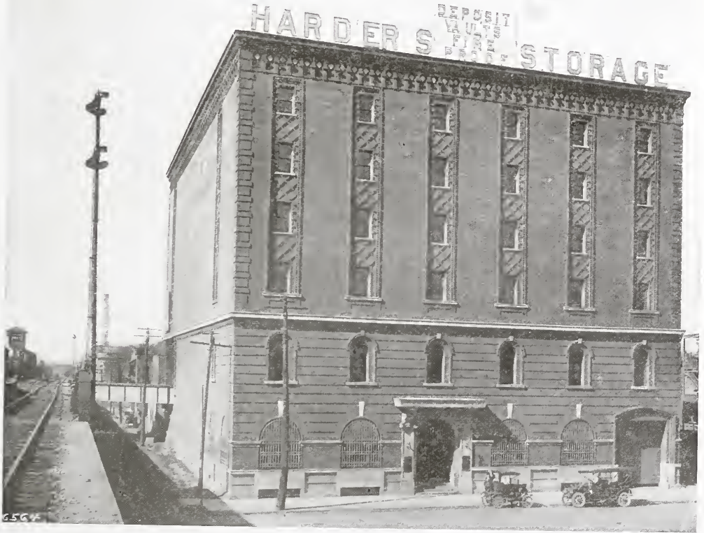
FIG. 4. HARDER'S FIREPROOF WAREHOUSE—CALUMET AVENUE BUILDING. Chicago, Ill.
