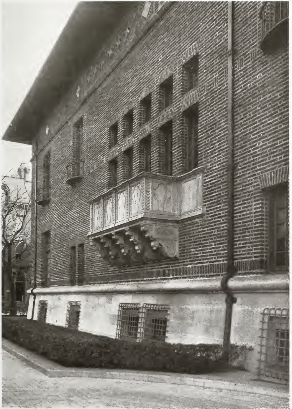
A DETAIL OF THE RESIDENCE OF HON. JOHN R. McLEAN, WASHINGTON, D. C.
