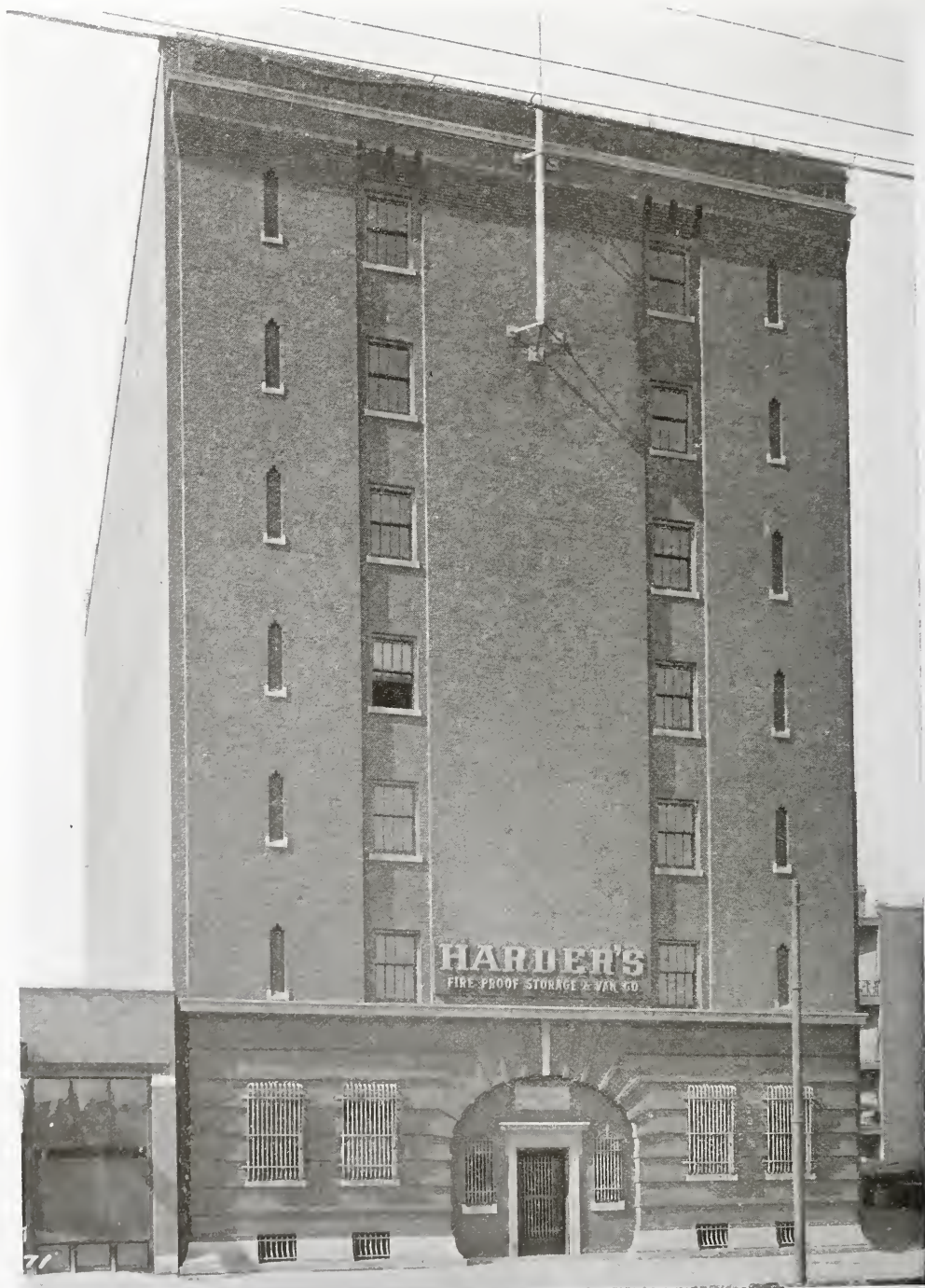
FIG. 3. HARDER'S FIREPROOF STORAGE AND VAN CO. BUILDING. Chicago, Ill. Horatio R. Wilson, Architect.
