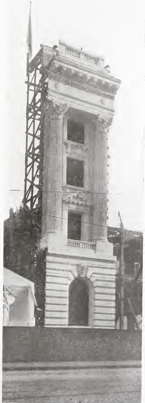
Full Size Model (Executed in Staff)—U. S. Post Office, Custom House and Court House. Cleveland, Ohio. Arnold W. Brunner, Architect.
