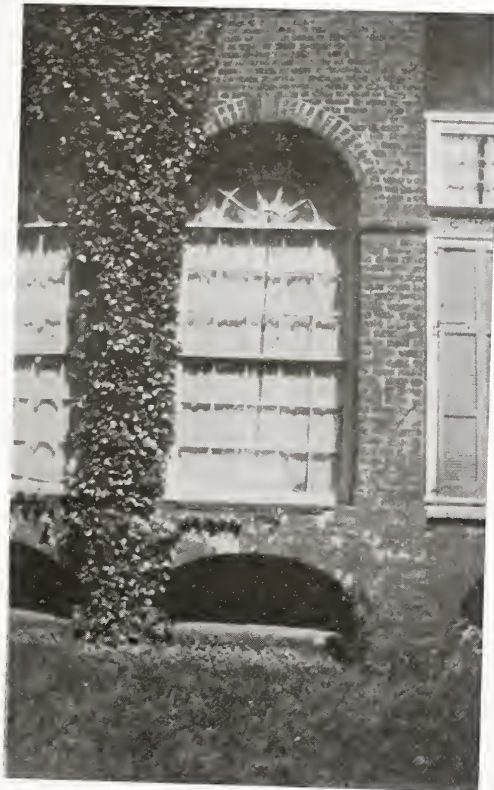
Window and Basement Ventilation, "Monticello."
