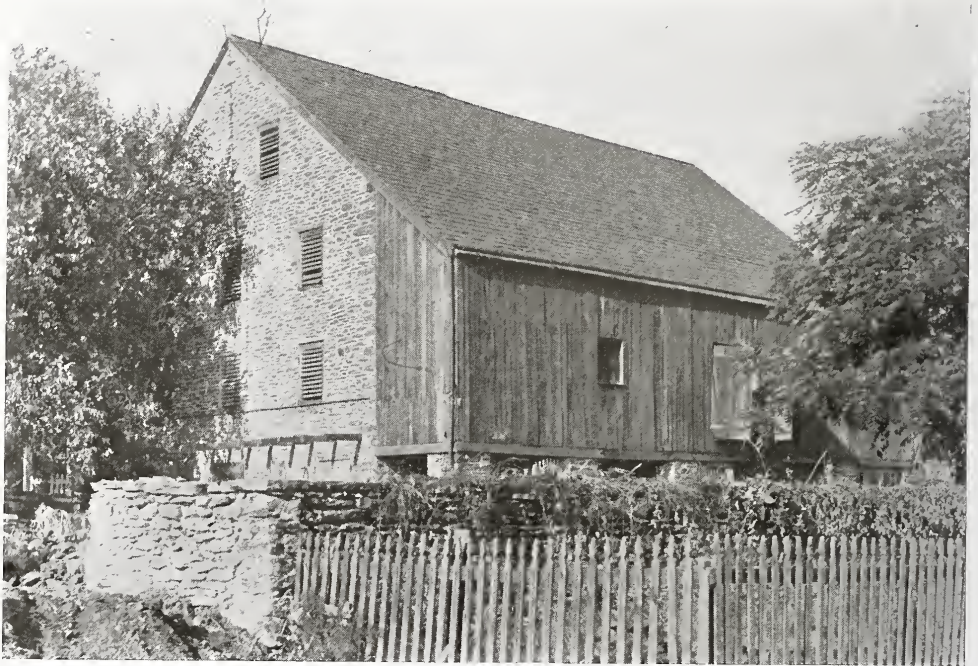
BARN FROM WHICH RESIDENCE OF MANTEL FIELDING WAS BUILT.
