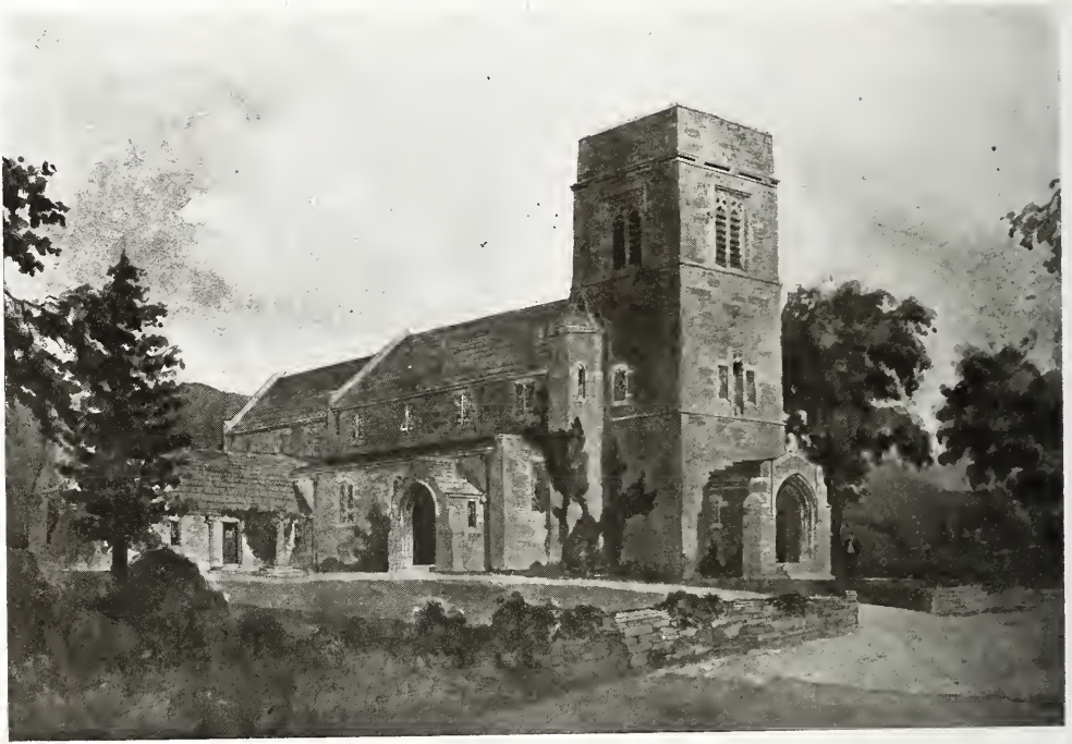
ST. MARKS' CHURCH, MT. KISCO, N. Y. New York Office, 1909.
