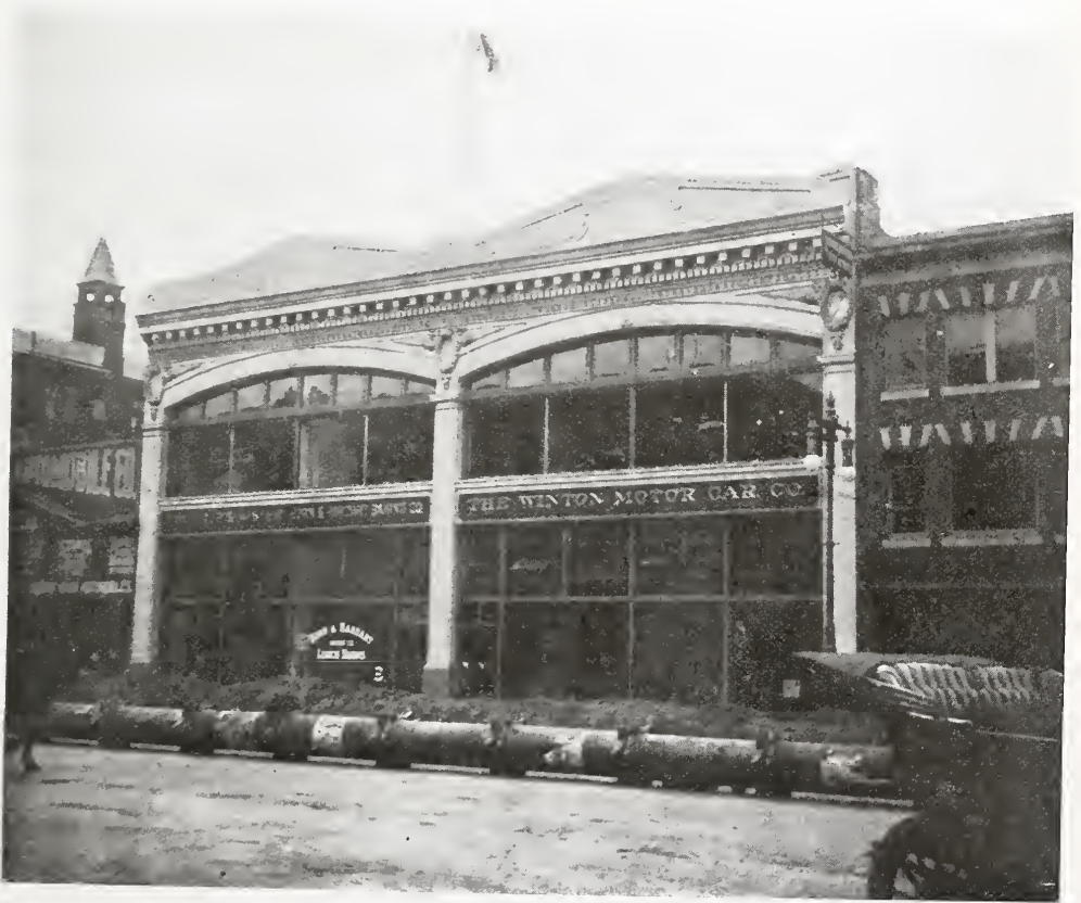
FIG. 1. MODERN CONCRETE BUILDING USED AS A GARAGE.
