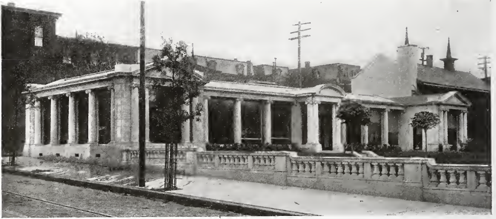
GREENHOUSE—THE A. E. BURK RESIDENCE.
