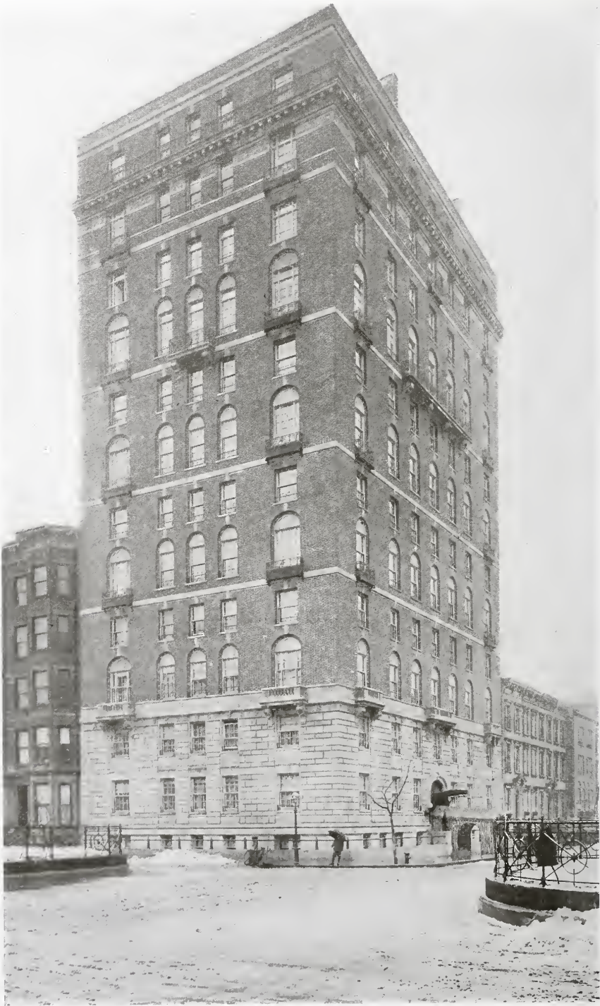
FIVE HUNDRED SIXTY-THREE PARK AVENUE. New York City. Walter B. Chambers, Architect.
