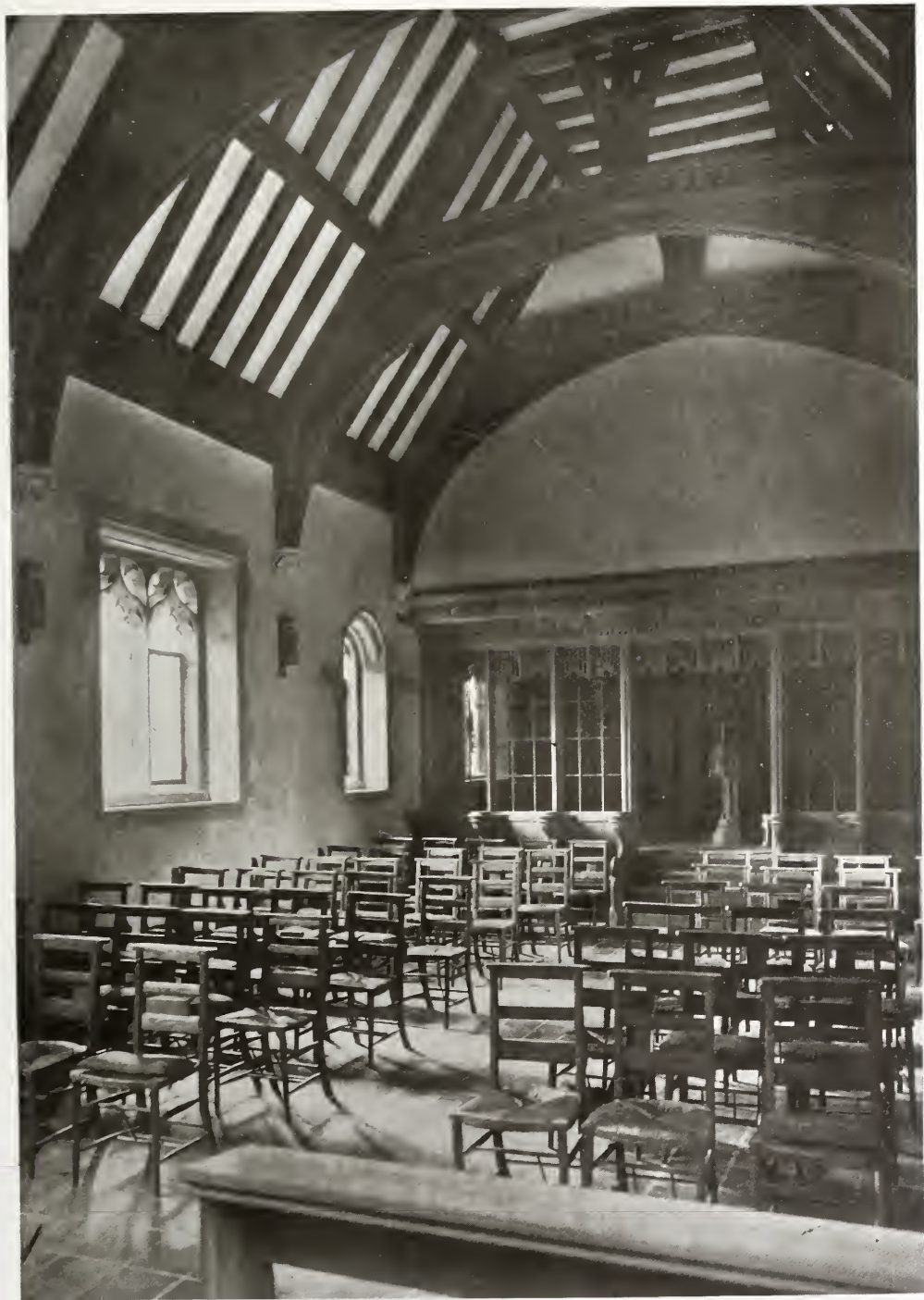
THE CHAPEL, ST. PAUL'S CHURCH, NEW HAVEN, CONN. New York Office, 1910.
