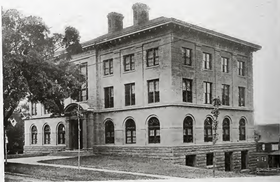
WILBUR FISK HALL (1903-4), WESLEYAN UNIVERSITY. Middletown, Conn. Charles A. Rich, Architect.
