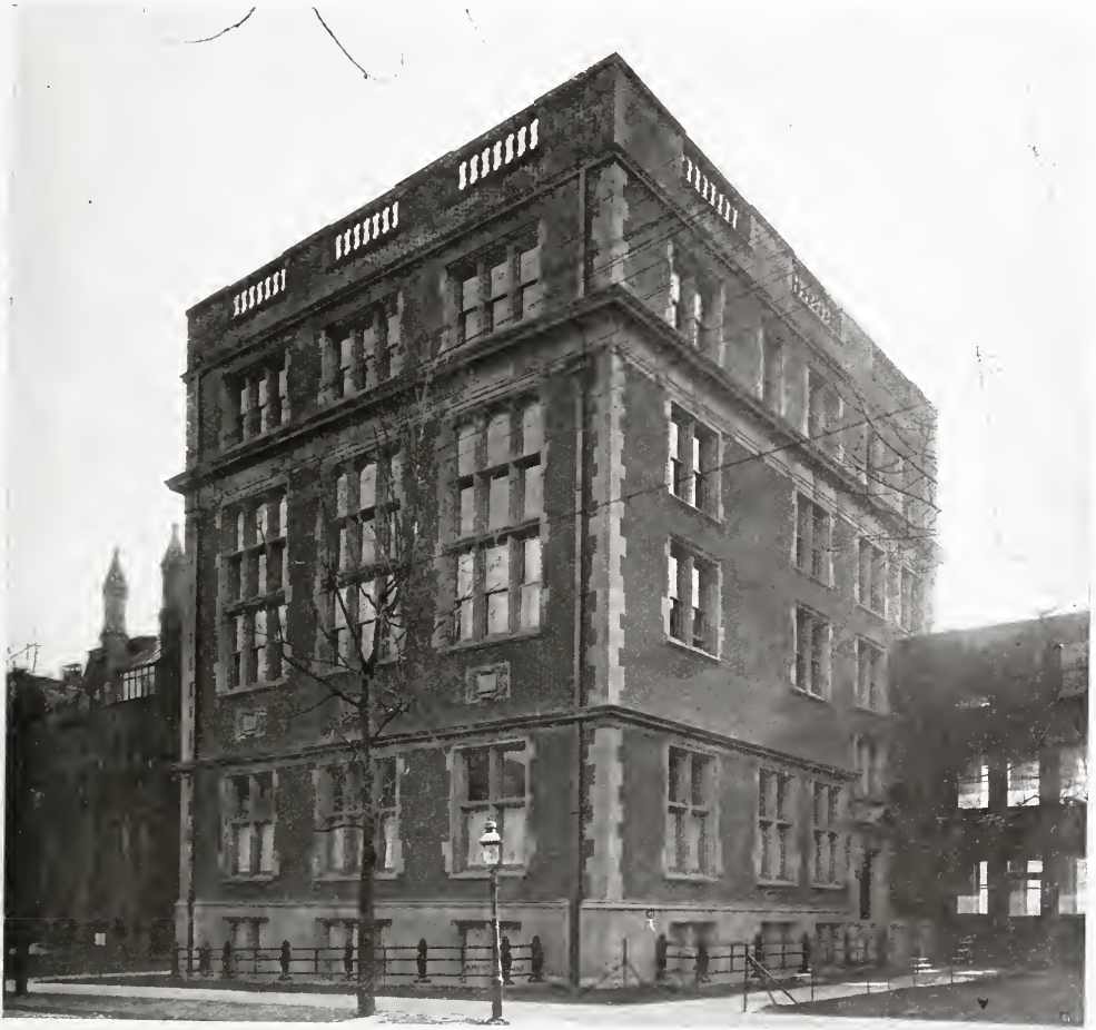
NEW HOSPITAL BUILDING—UNIVERSITY OF PENNSYLVANIA.
