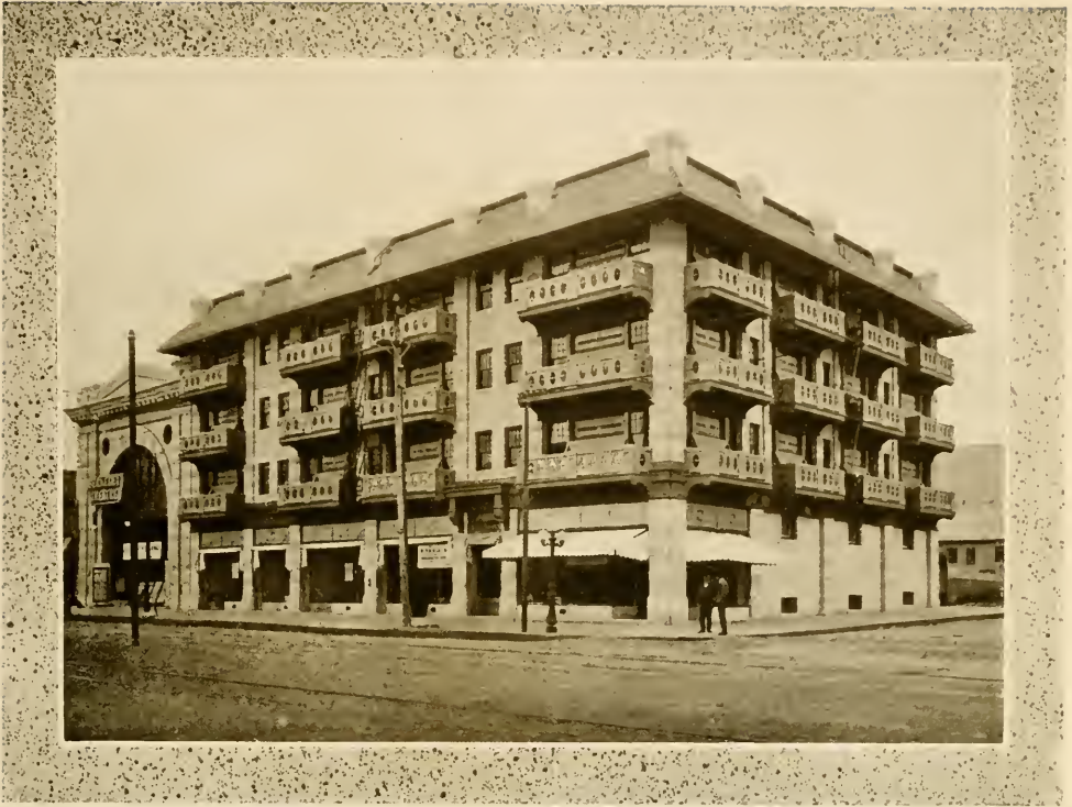
THE HANDSOME NEW BERKELEY THEATRE BUILDING, SITUATED AT SHATTUCK AVENUE AND DWIGHT WAY
