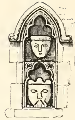
Blocked Spire-light, St. Hilary.
