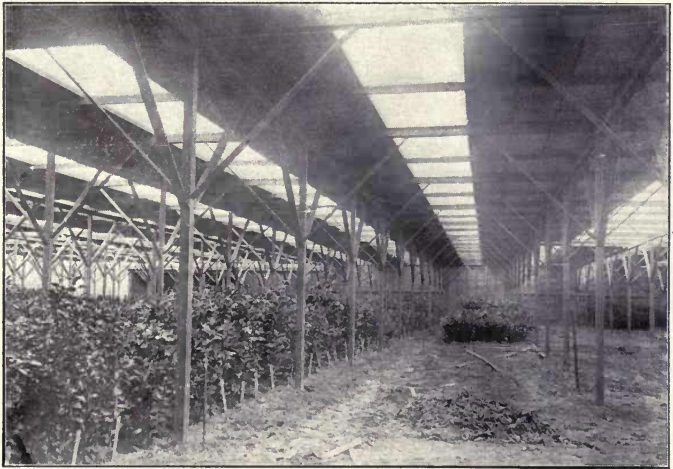
Fig. B. Interior view, showing construction. Shed erected by G. L. Taber, Glen Saint Mary Fla.
