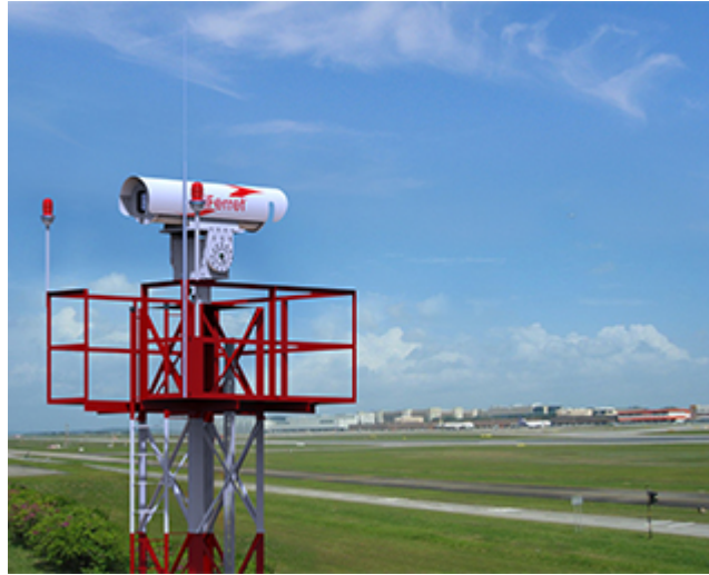
Figure 6. Static position iFerret camera overlooking airfield. Source: iFerret (2015).
