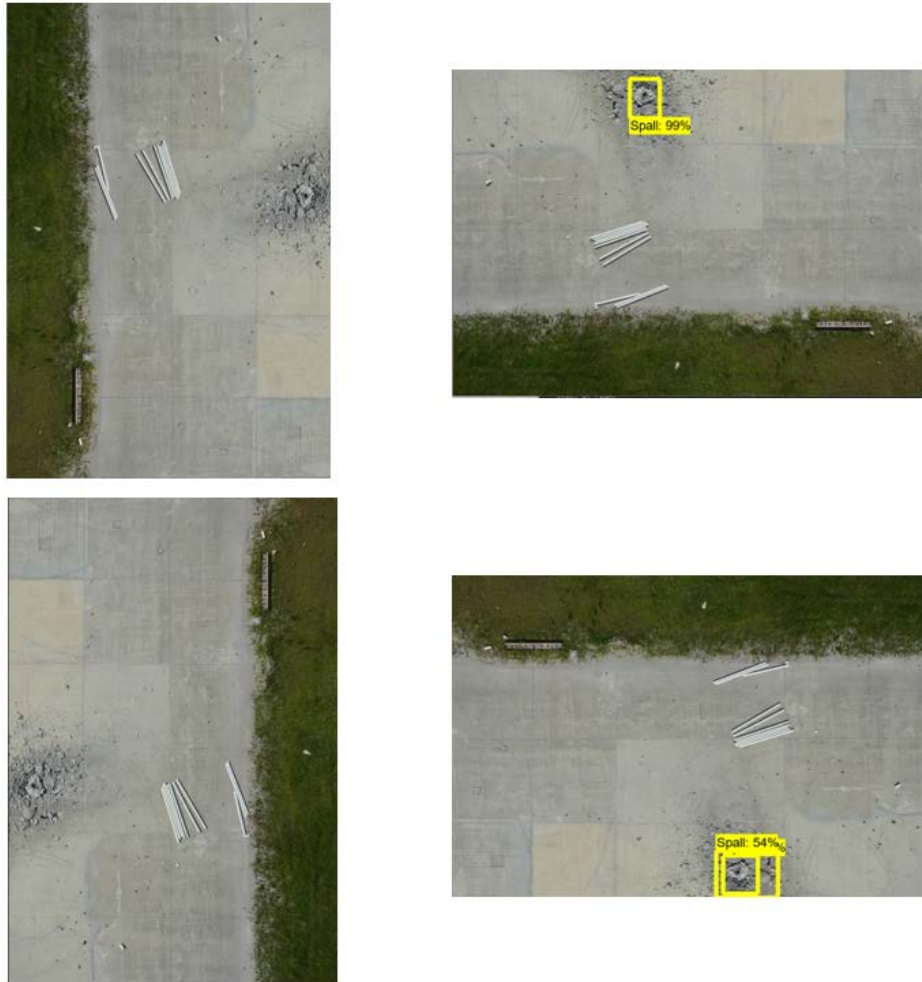
Figure 35. Example of differing detection results of the same image rotated on all four axes.
