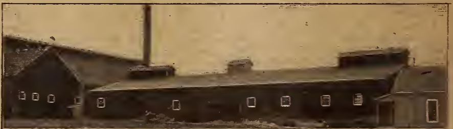
PARTIAL VIEW CANEY GLASS COMPANY'S PLANT. Roofed with 55,000 square feet Amatite
