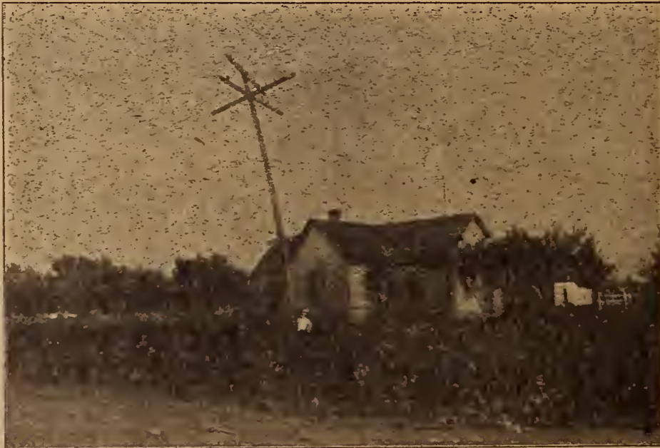
This pole, located at a cross roads, carries nineteen telephone wires, each wire being connected with nine to fifteen farm homes. Five years ago there was not a telephone in this locality, except the Long Distance in town. This shows how farmers appreciate a really good thing. Free rural delivery of mail and the telephone have brought the country into town—in close touch with all the world.
