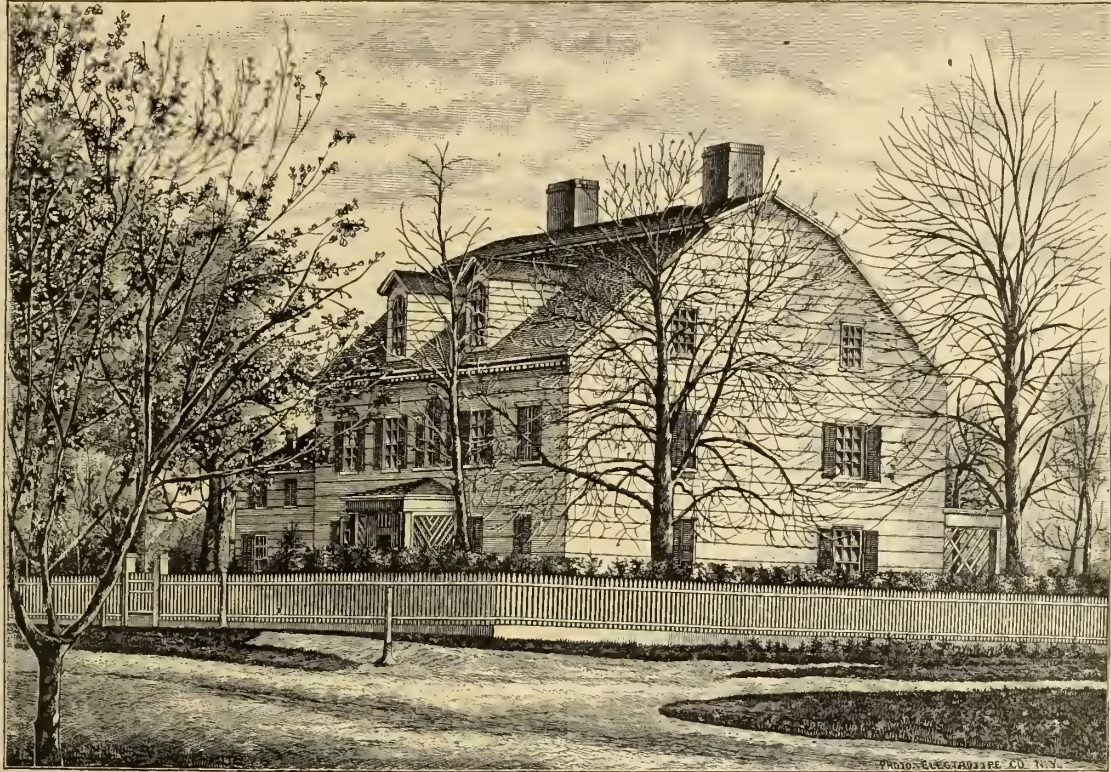
ST. GEORGE'S CHURCH RECTORY; BUILT 1793.
