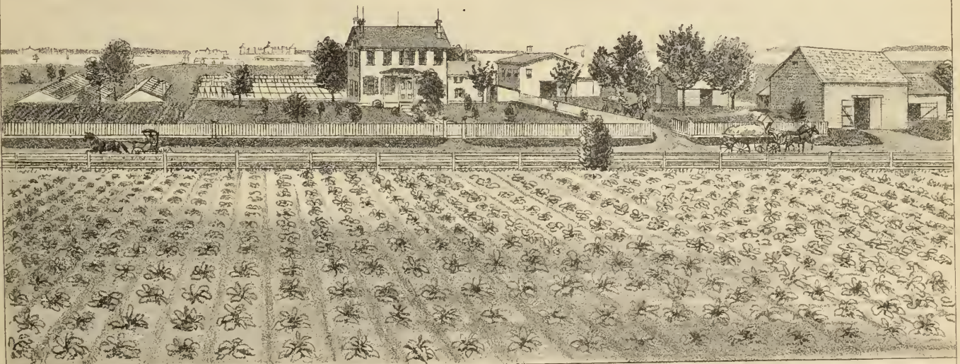
RESIDENCE OF JOHN B. HOPKINS, JAMAICA EAST, QUEENS CO., N.Y.
