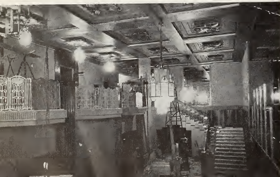
Reconstruction at the balcony (above). The walls proved strong enough, to support cantilever construction, thereby eliminating all posts. The wooden structure is scaffolding erected to increase workmen's speed.
