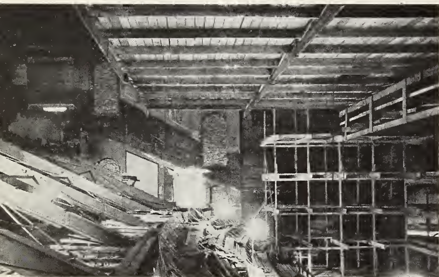
Reconstruction at the balcony (above). The walls proved strong enough, to support cantilever construction, thereby eliminating all posts. The wooden structure is scaffolding erected to increase workmen's speed.
