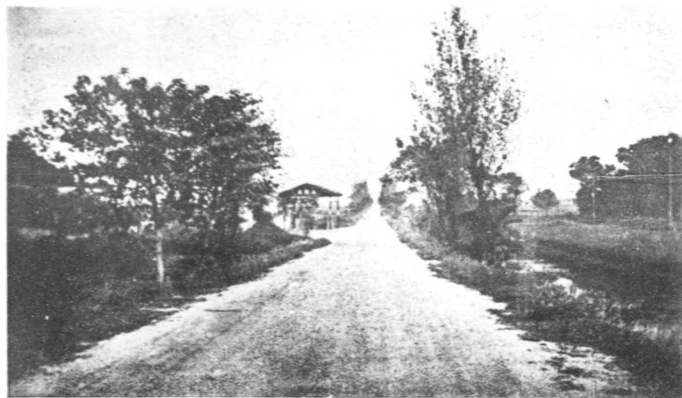
Clay Bound Macadam-by the penetration method-Chekiang, China.
