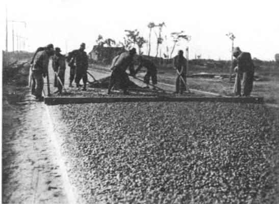
The cold laid bituminous pavement at Shanghai, showing condition under construction.
