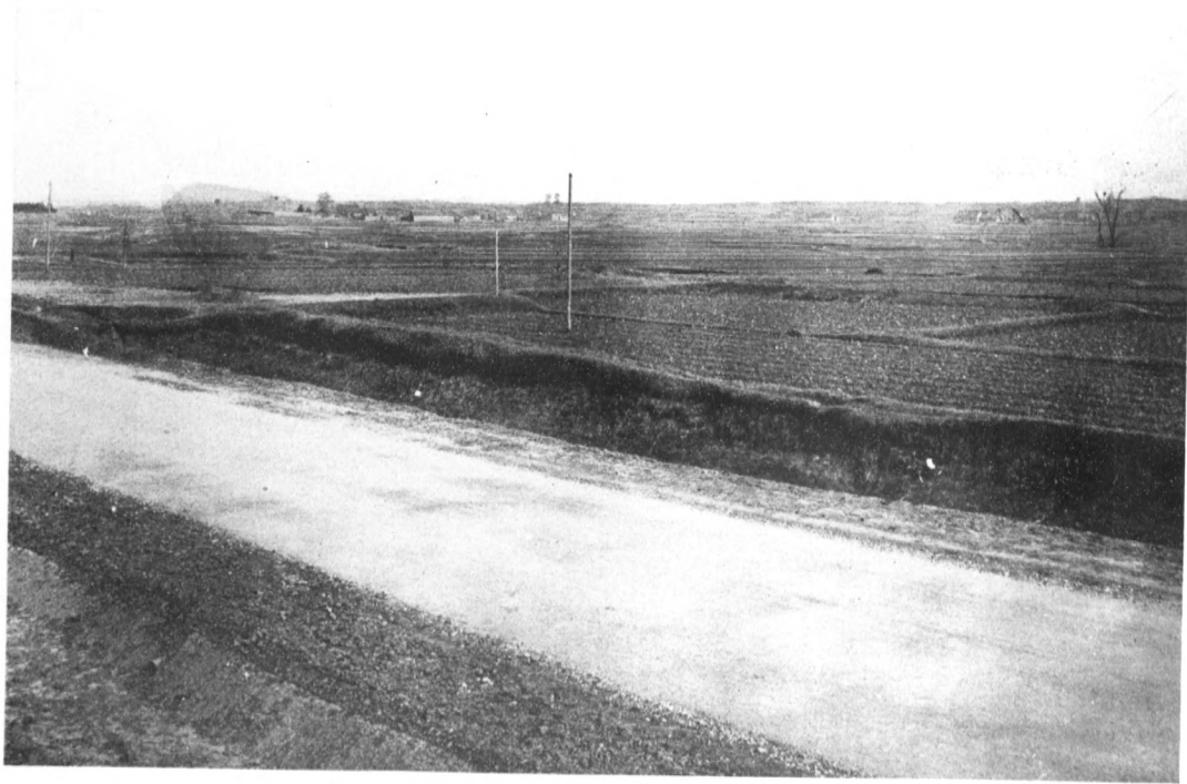
Clay Bound Macadam-by penetration method-Nanking, China
