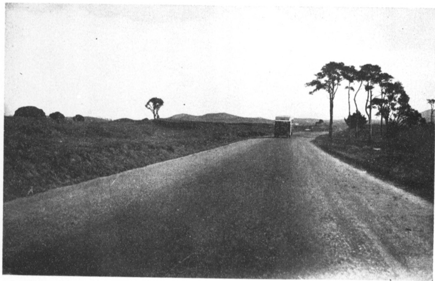
A 2.8 meter single coat bituminous surface treatment of a 5½ meter clay bound macadam.
