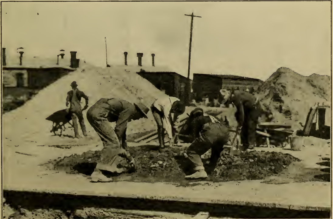
The entire mass is then turned thoroughly several times until every pebble or particle of broken stone is covered with sand-cement mortar and the whole mass is of uniform consistency.
