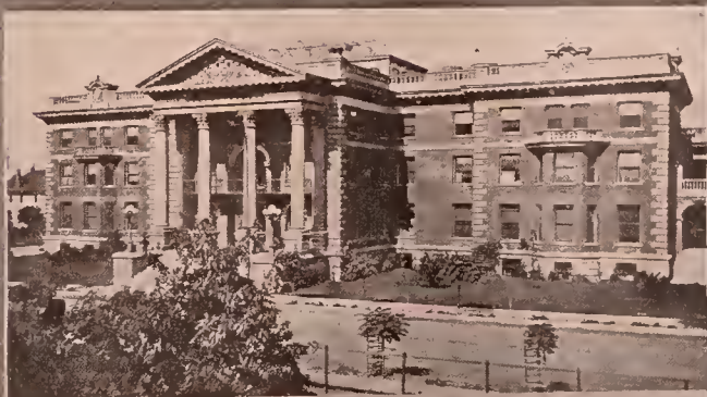
ANGELUS HOSPITAL, Los Angeles
