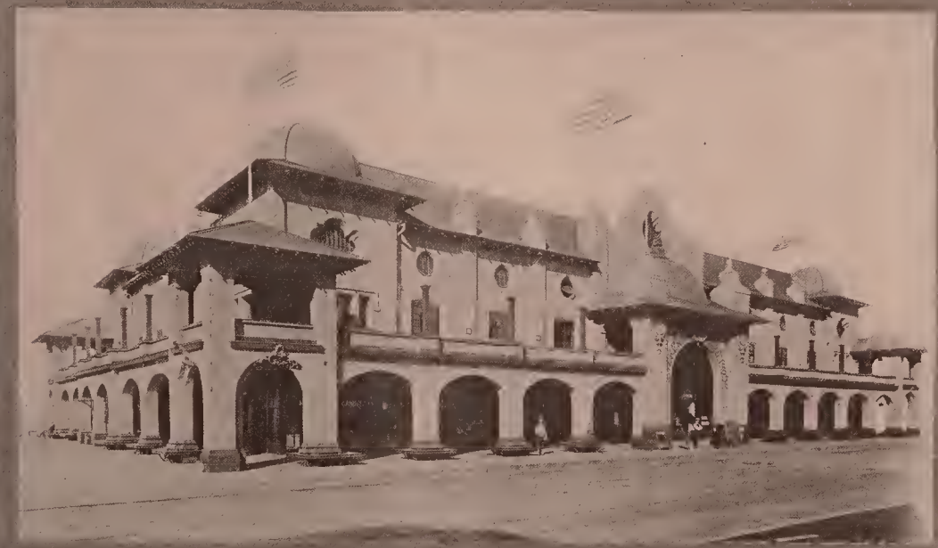
PAVILLION AUDITORIUM, REDONDO BEACH.
