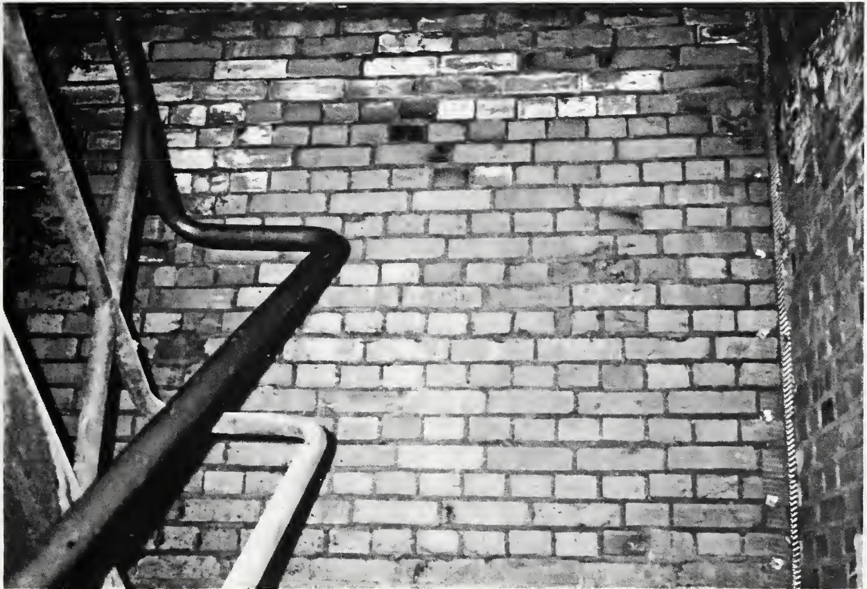
Figure 5.8.3. Good quality partition wall in stairwell
