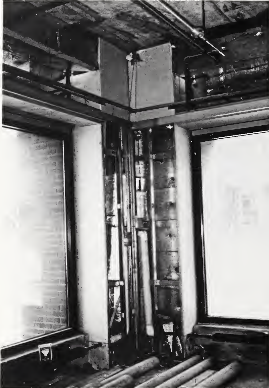
Figure 5.6.12. Insulation in northeast corner in second story
