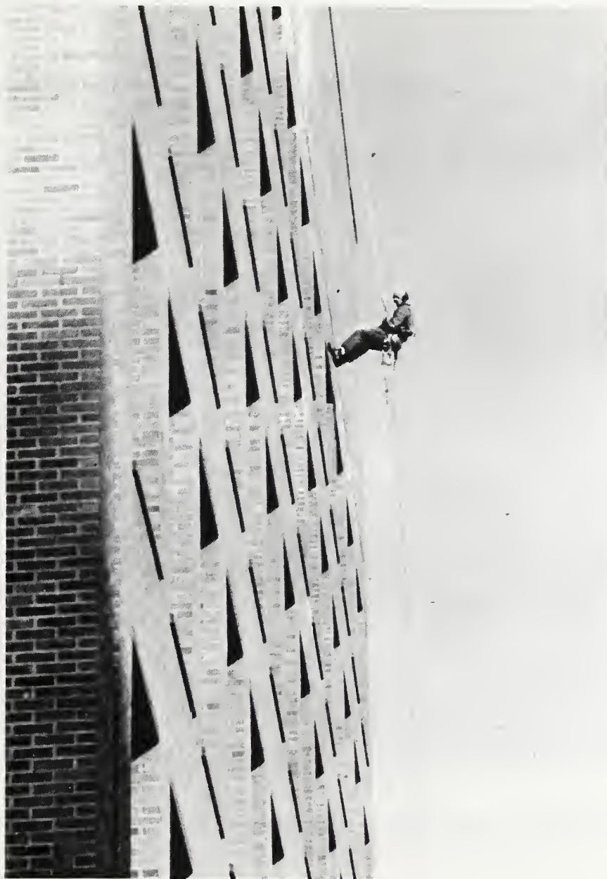
Figure 5.6.1. Examination of exterior walls using technical mountaineering equipment
