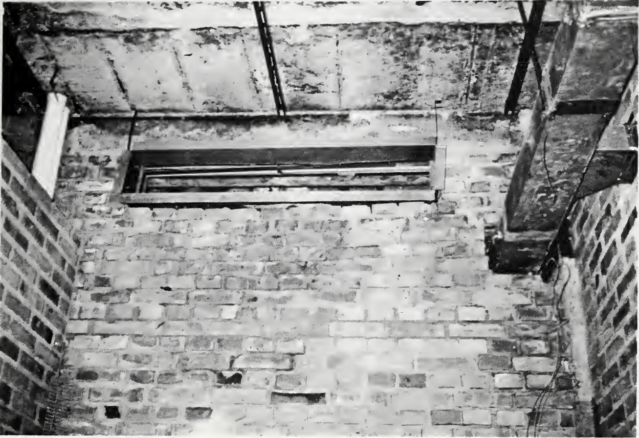
Figure 5.8.5. Duct penetration in partition wall
