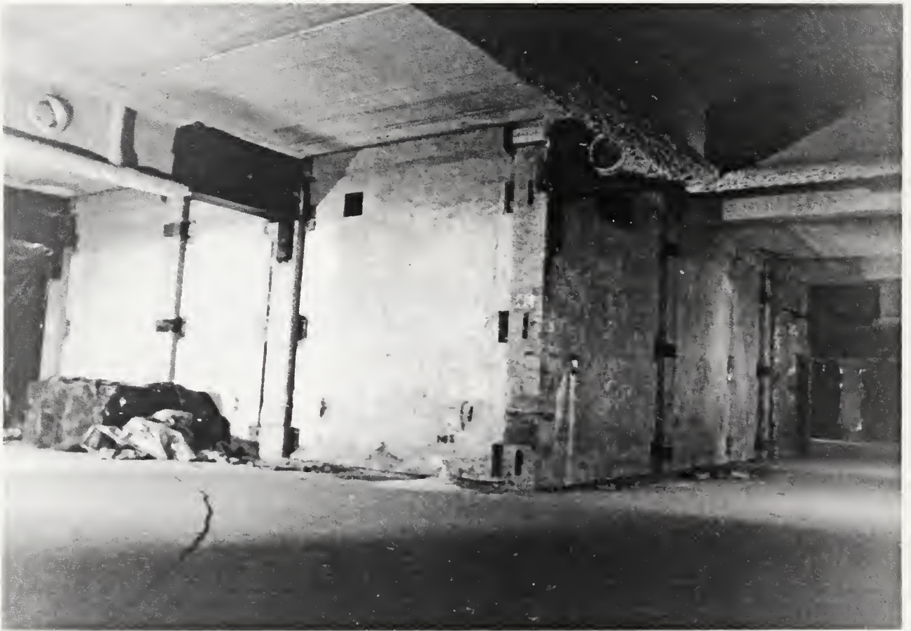
Figure 2.3.19. View showing shear walls
