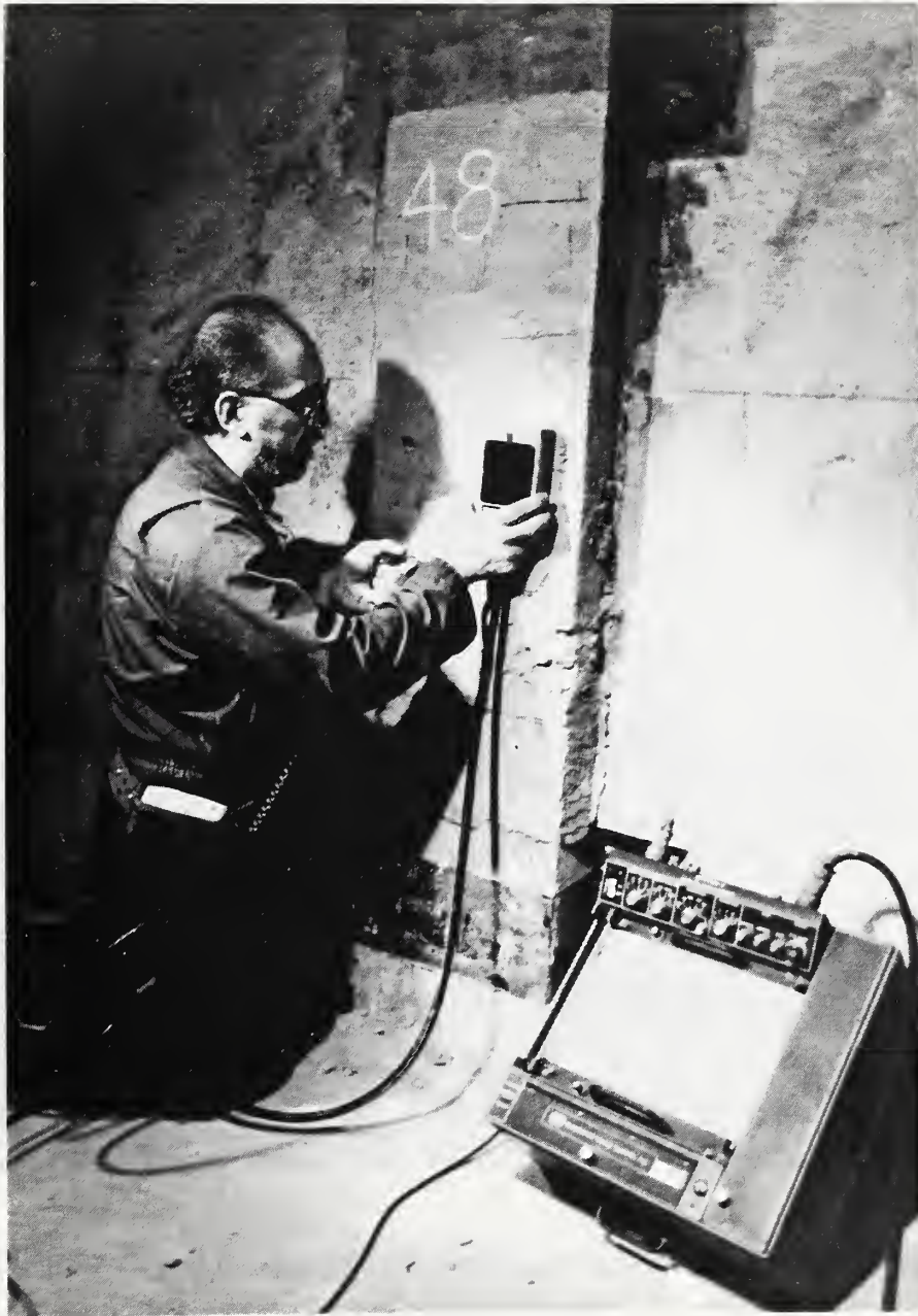
Figure 5.3.3. Radar inspection of column
