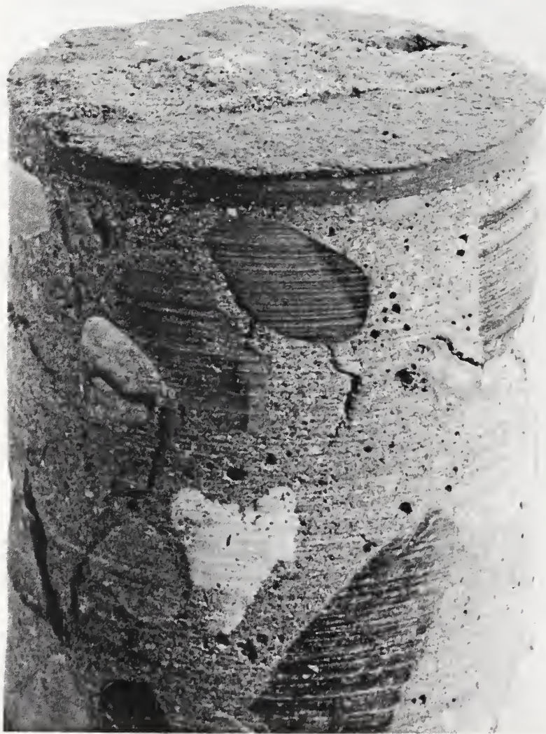
Figure 5.6.14. Core from eighth story wall showing bond of concrete to brick
