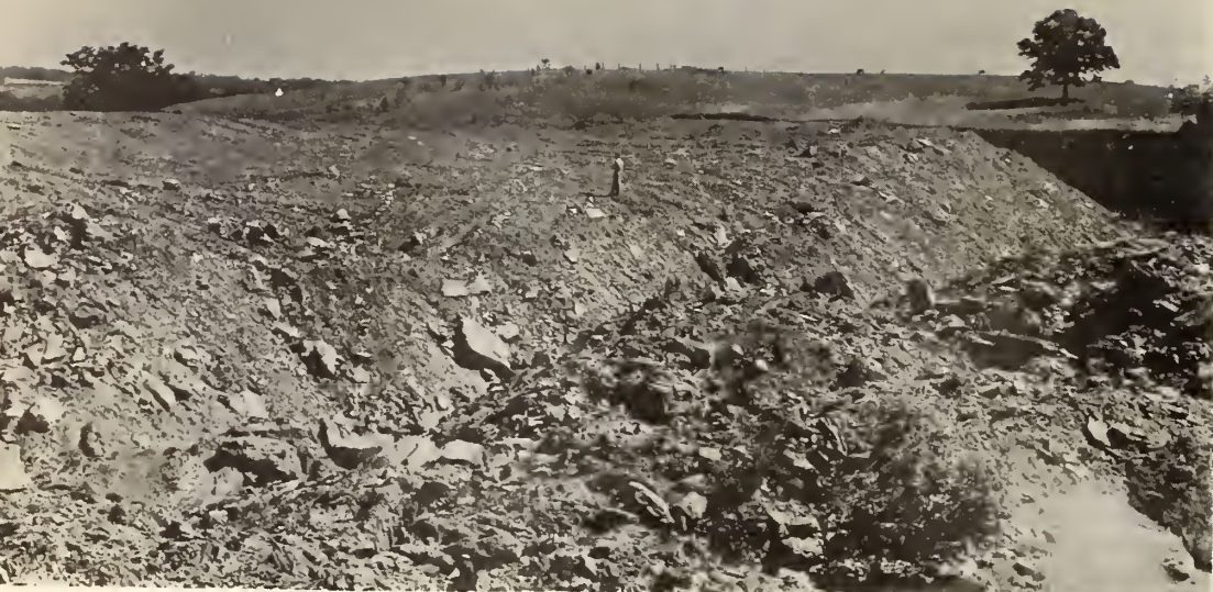
Figure 2.--Graded (left) and ungraded (right) No. 7 banks before planting.
