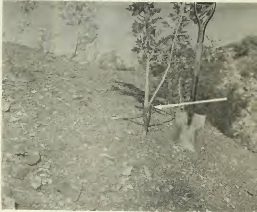
Figure 12.--In 10 years several inches of soil have eroded away from near the top of this No. 5 bank. Arrow shows ground line at time of planting.
