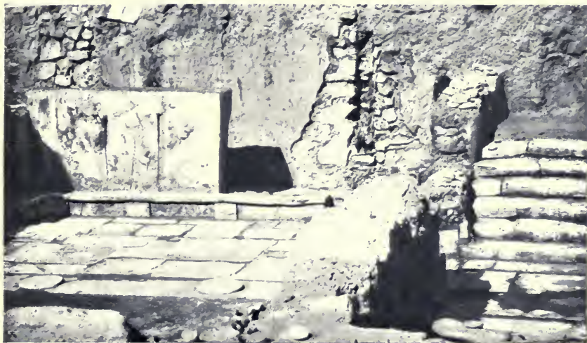
FIG. 24.—STAIRCASE LEADING FROM THE UPPER FLOOR TO THE PRIVATE APARTMENTS.
