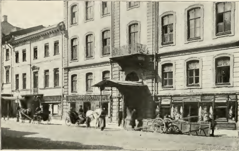
THE CHANCELLERY OF THE U. S. EMBASSY IN THE MILLIONNAIA
