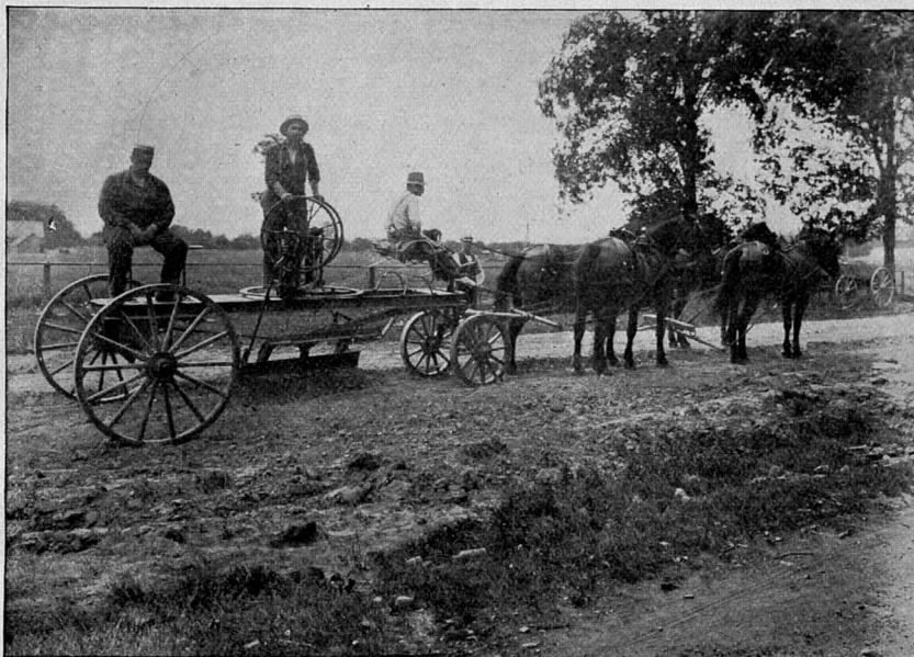
FIG. 1.—WORKING THE ROAD MACHINE.
