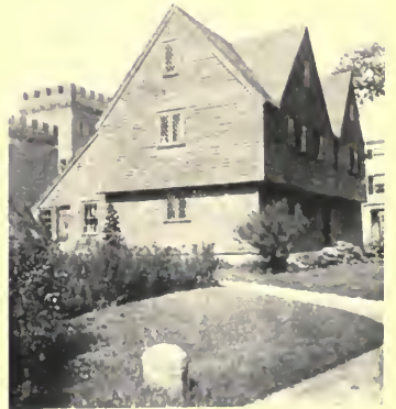
AN OLD HOUSE BUILT IN 1684 SHOWING GABLES, OVER-HANGING STORY AND THE LEAN-TO CHARACTERISTIC OF THE FIRST PERIOD OF SALEM ARCHITECTURE. NOW IN THE GROUNDS OF THE ESSEX INSTITUTE, SALEM.
