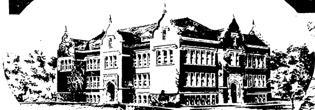
The High School in course of erection.
