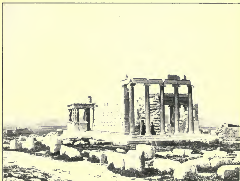
ERECHTHEUM FROM THE SOUTH-EAST.
