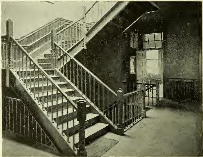
CORRIDOR ON THE SECOND FLOOR.
