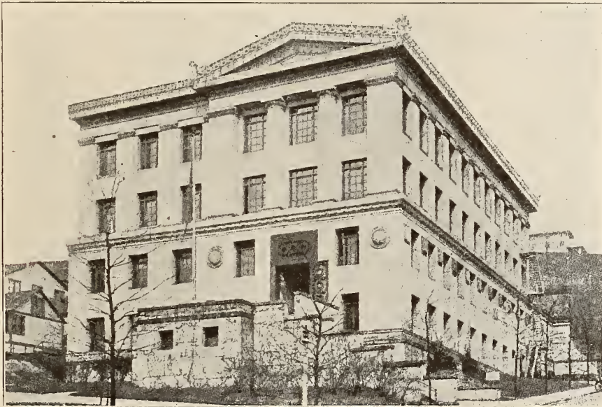
Headquarters of the Public Service Department
