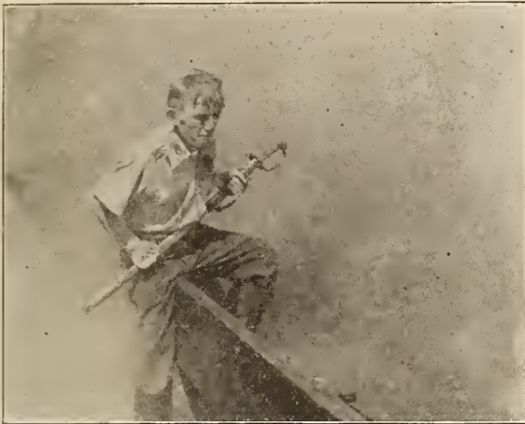
Johnny Ring Crossing the Burning Bridge
