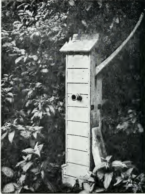
THE SEWAGE PUMP
