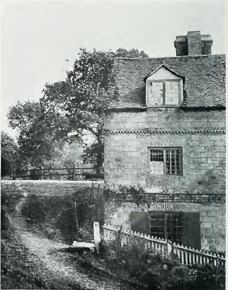
THE MILL-HOUSE, ENTON
