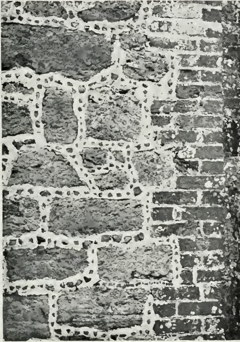
WALL WITH GARNETED JOINTS
