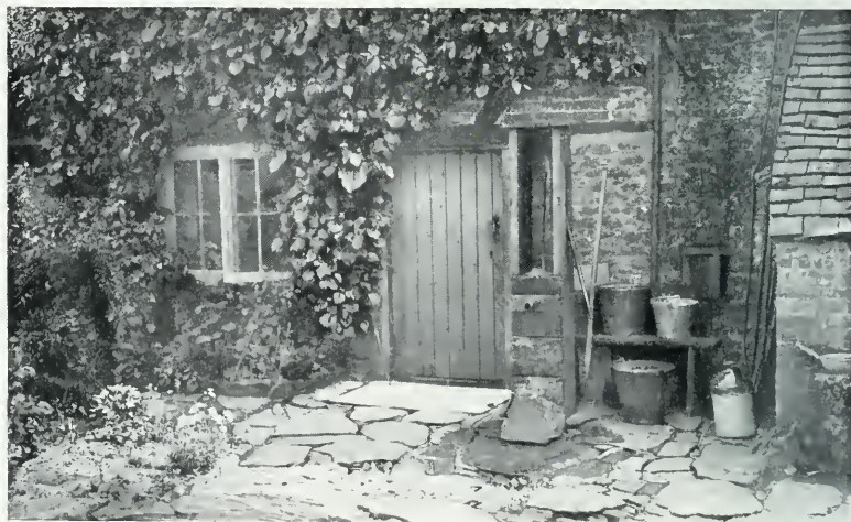
STONE PAVING AT COTTAGE ENTRANCE
