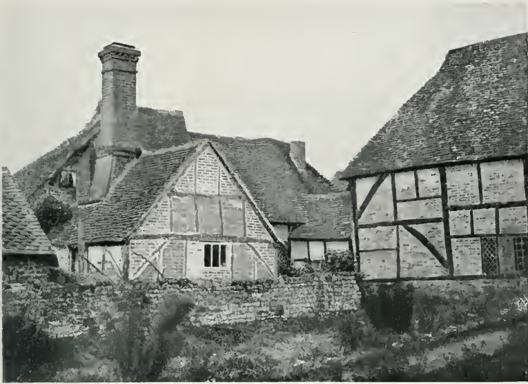
TIMBER-FRAMED COTTAGES, ELSTEAD
