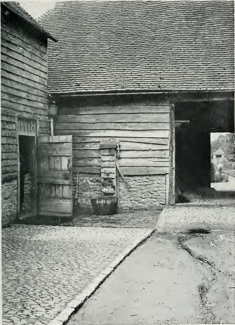
IRON-STONE PITCHING WITH BARGATE KERB
