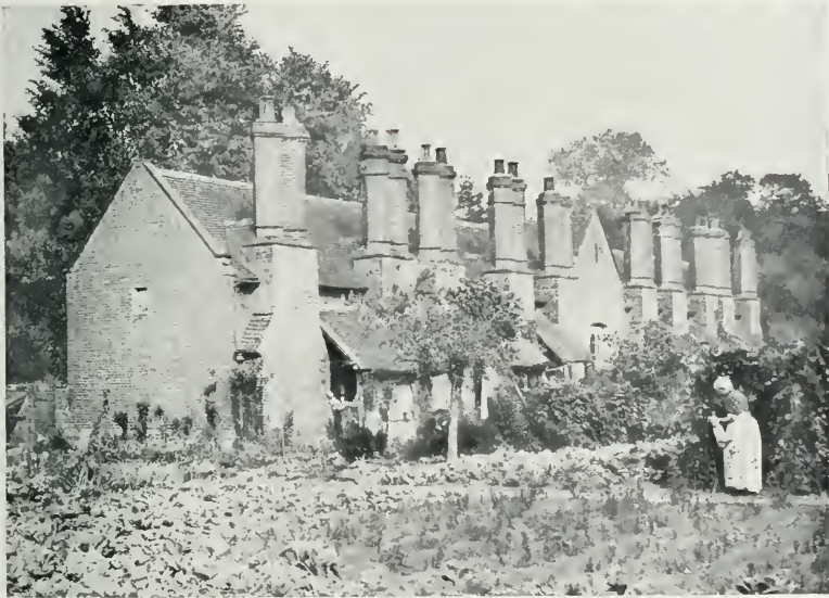
BACK OF WYATT'S ALMSHOUSES
