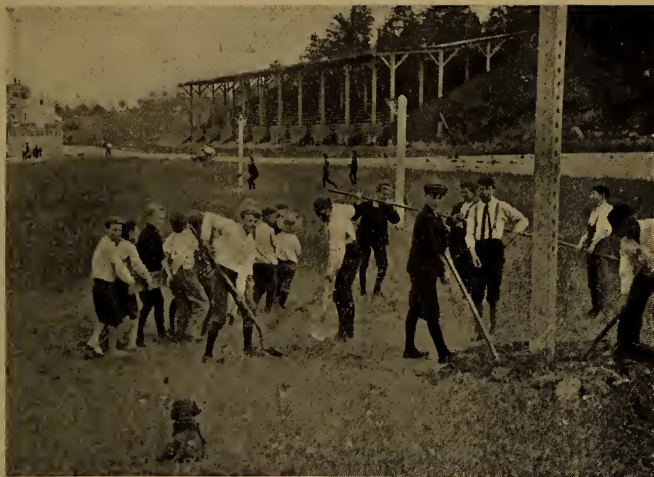
THE EQUIPMENT OF A PLAYGROUND. Page 39
