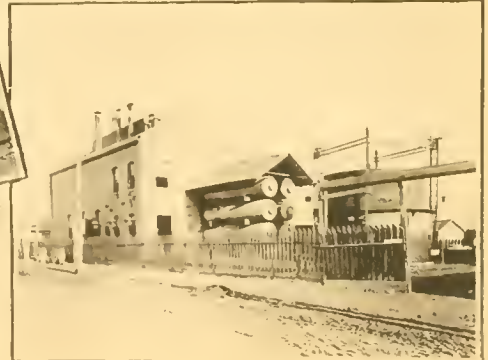
1000 PINTON POWER PLANT
