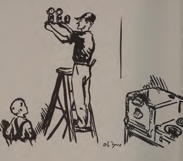
button at the right of the front door. When the button was pushed a chime rang. He put a pushbutton to the right of the back door. When this button was pushed a buzzer sounded. One could tell by the sound whether a person was at the back door or the front door.
