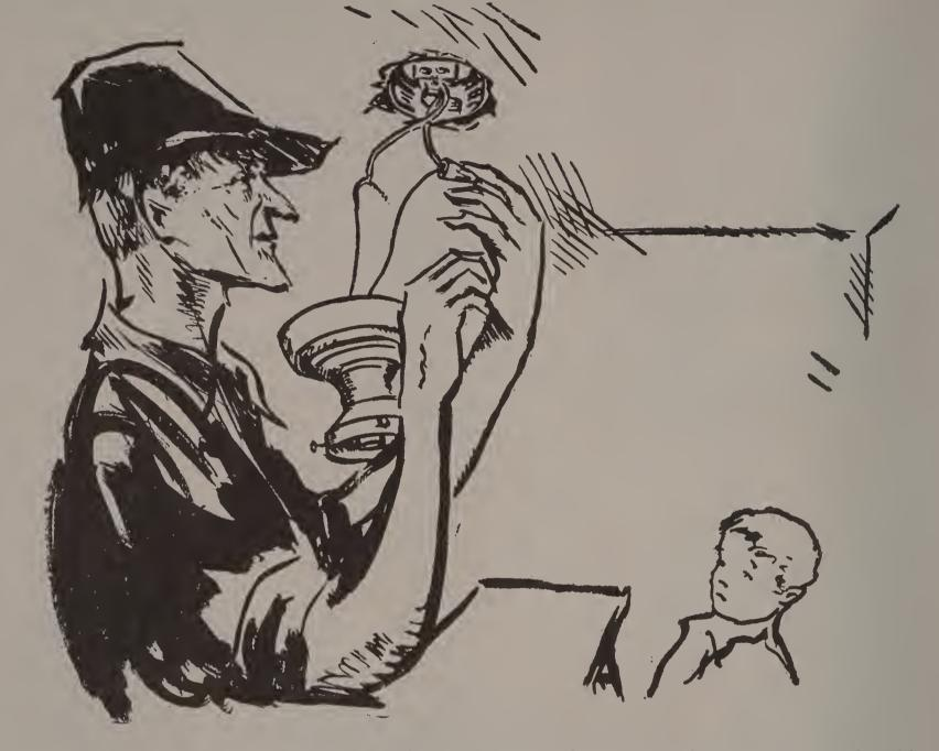
Sparks next installed the switches, plugs, and light fixtures. Where he connected the wires from the fixture to the wires in the box he covered the joint with a nipple. A nipple is a piece of hard rubber that looks like Mother's thimble.
