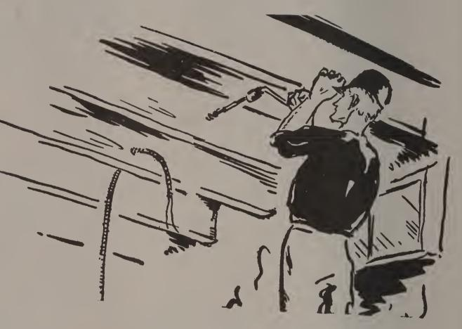
current would flow into the ground. It would not hurt anyone. Where there was to be an outlet he cut his wires and left them hanging. Later he would put small metal boxes at each place. When Sparks spliced a wire he soldered the joint and covered it with friction tape.
