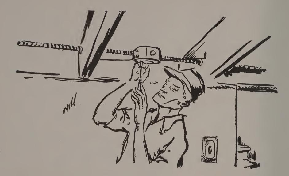
Sparks fastened little metal boxes at each outlet. He brought the cable and wire into each box through holes in the side of the boxes. The boxes for switches and plugs were square. The boxes for ceiling lights were round. The switches or ceiling lights would cover the boxes when the house was finished.
