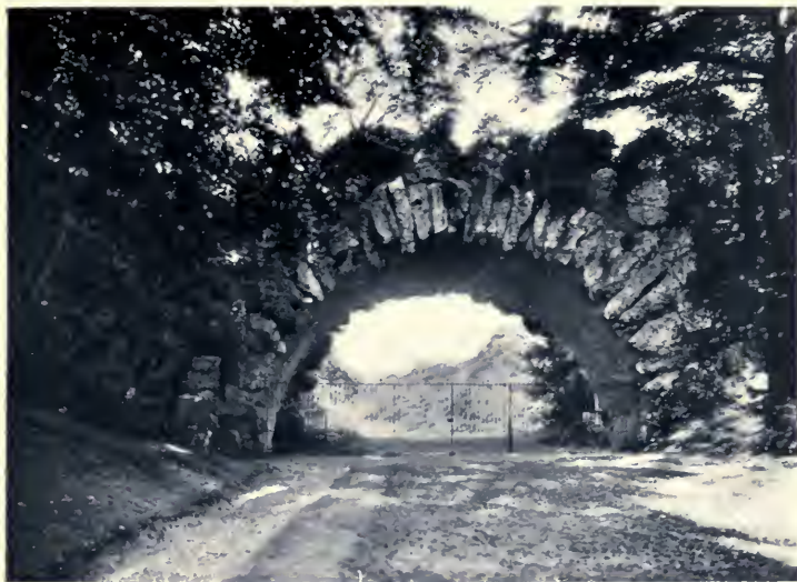
ARCH CARRYING THE ROAD, PARK PLACE.
