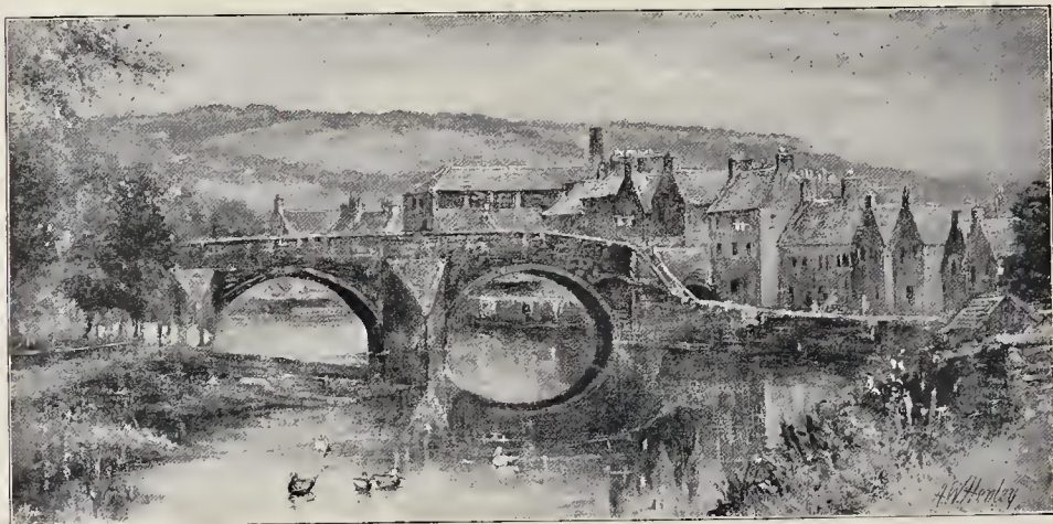
Nungate Bridge, Haddington.
