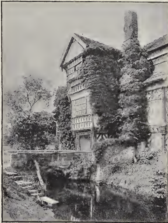
Entrance Gateway and Bridge. From a Photograph by R. Keene.
