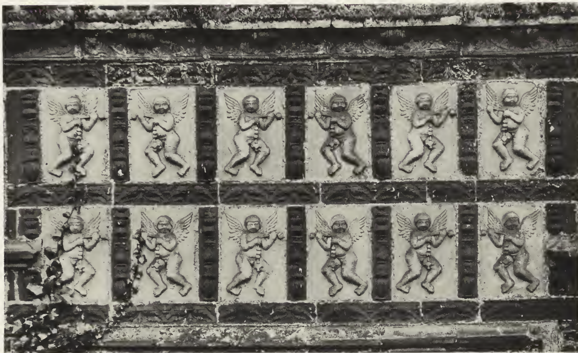
TERRA-COTTA WORK OVER DOOR LEADING TO GREAT HALL SHOWING AMORINI DIVIDED BY A BALUSTER DESIGN IN THE STRING COURSE ABOVE APPEARS THE "TUN"—FOR WESTON
