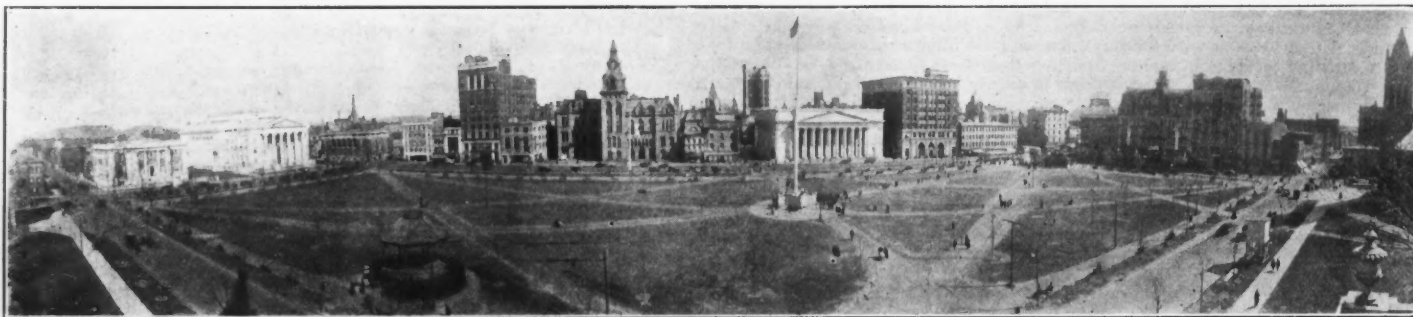
The two beautiful structures to the left are the Public Library and the Superior Court. Modern office buildings, including the Chamber of Commerce and the old City Hall, follow in order, and the magnificent new Post Office and Federal Building—a veritable "Greek Temple"—which has but recently been completed, give to this city center a distinctiveness and impressiveness hard to match. The buildings to the right are office structures and retail establishments.
