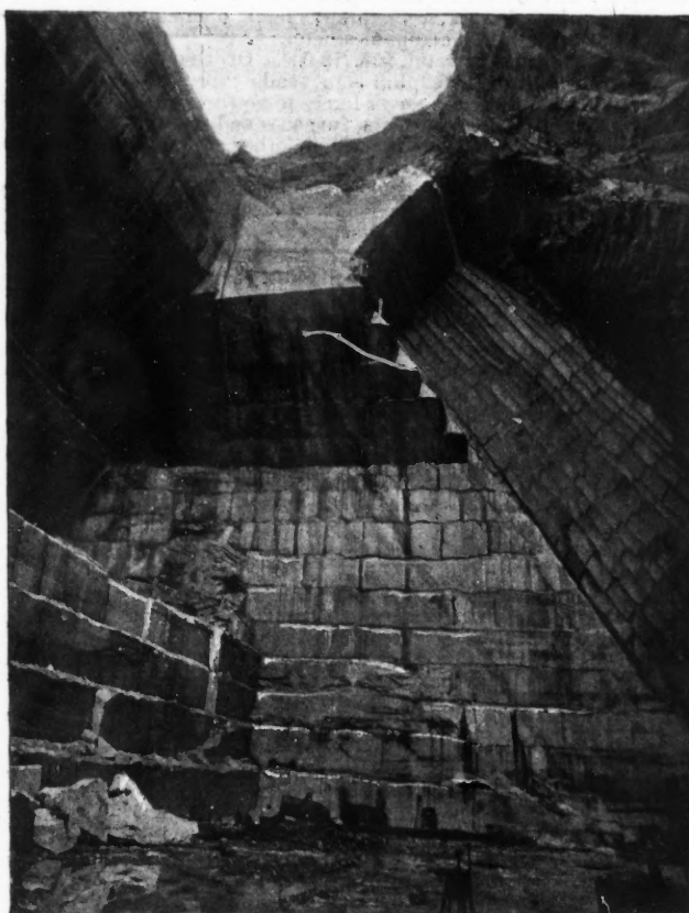
SHELDON QUARRY, WEST RUTLAND, VT., SHOWING HAND WORKINGS ON THE RIGHT. DEPTH TO THIS FLOOR 150 FEET.
