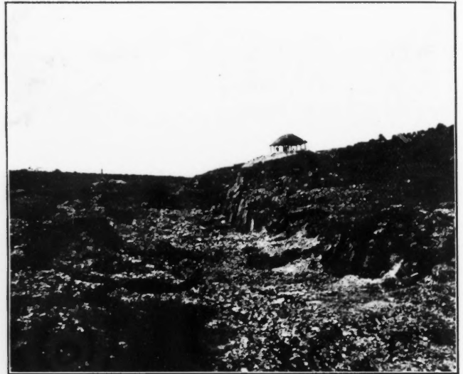
NATIVE TRENCH, KOLWEZI COPPER MINE—ORE FULL WIDTH OF TRENCH
