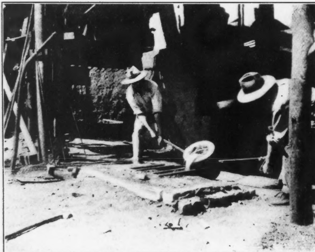
CASTING COPPER FROM GALVANIZED-IRON BUCKET LINED WITH CLAY
