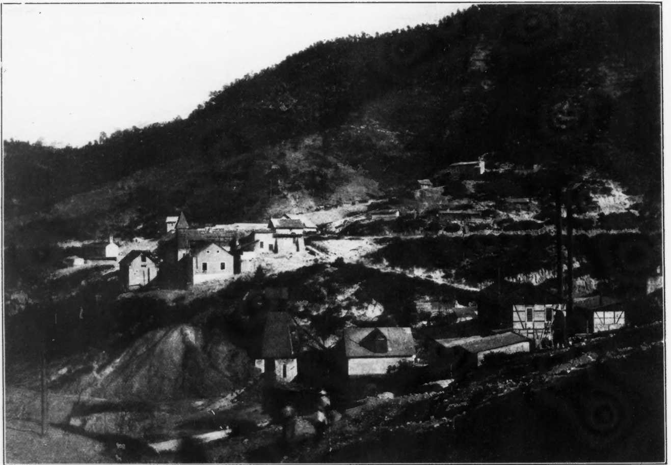
THE PROMONTORIO MINE LOOKING EAST—REFUGIO SHAFT, SAN JOAQUIN DUMP, ADMINISTRATION BUILDING, POWER HOUSE
