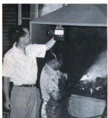
Tests of air velocities made at the worksite make sure that the engineering control of poisonous vapors is adequate. Where a localized exhaust system, as shown, is provided, each process needs a specific air velocity at the point of air entry.
