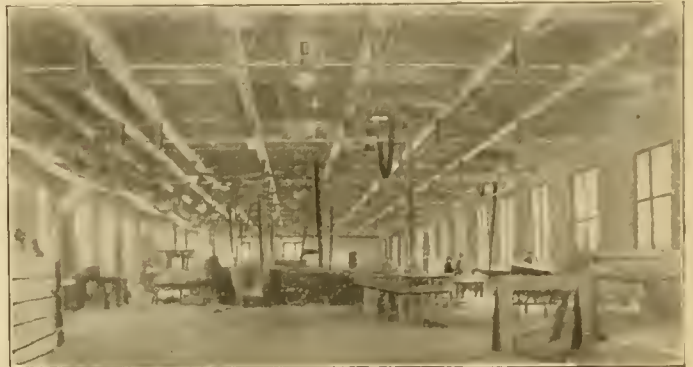
Planing Mill from North End.
