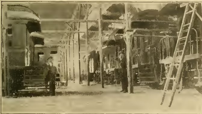
Passenger Car Paint Shop Showing Stagings.
