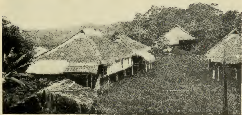
PLATE 57.—Cayapa houses and village. Top: Typical dwelling along river. Center: Unfinished house showing roof structure. Bottom: Chief's house at Sapayo Grande. (After Barrett, 1925.)
