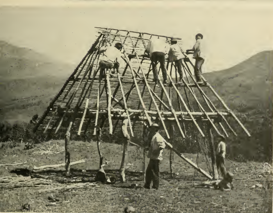
PLATE 39.—Hip-roofed house of the Guaymí. Top: Completed. Bottom: Framework. (Courtesy Frederick Johnson.)
