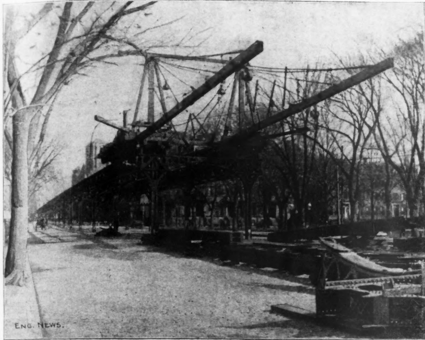
FIG. 3.—VIEW SHOWING ERECTION IN PROGRESS ON WASHINGTON ST., NEAR WORCESTER ST.
