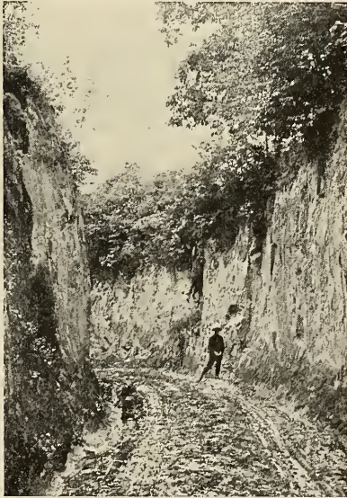
FIG. 62.—A road through a deposit of deep loess along the lower Illinois River. The deposit is 30 to 50 feet deep. The vertical walls are characteristic.
