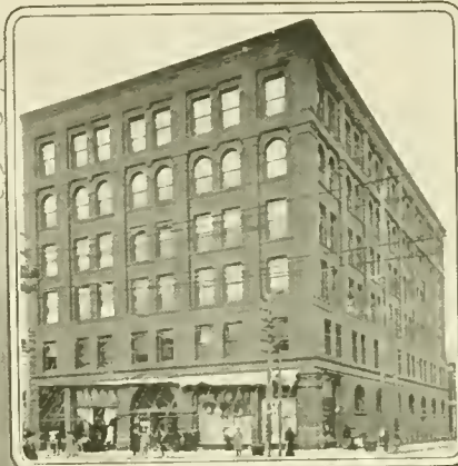
Downing Building-Ninth & State Sts
