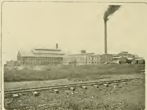
Erie City Iron Works
