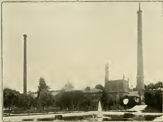
North view of Waterworks Pumping Station.
