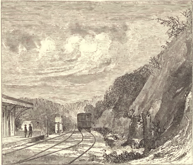
CUTTING ON THE SÃO PAULO RAILWAY, SHOWING DRIFT LYING ON DECOMPOSED ROCK.*
