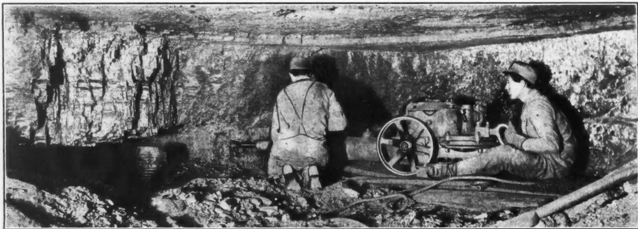
PNEUMATIC COAL PUNCHER IN OPERATION IN MINES OF THE BERWIND-WHITE COAL COMPANY, WINDBER, PENN.
