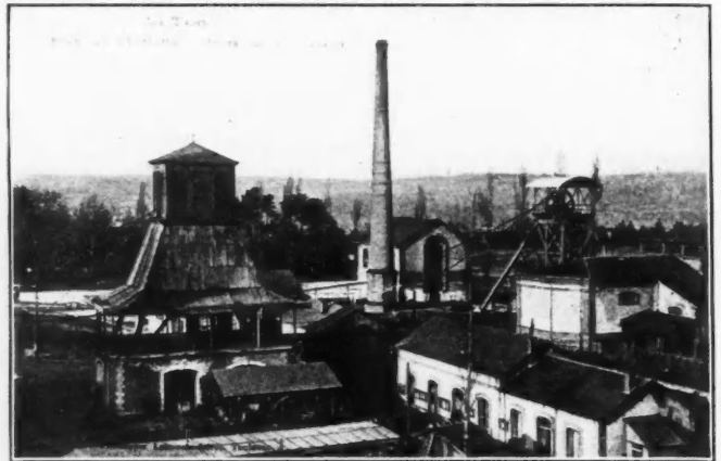
FIG. 2. LA GRILLATIE WAS ONE OF THE FIRST PLANTS BUILT
