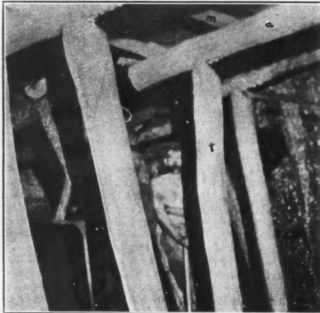
FIG. 3. THE TIMBERING IS NOT ALWAYS PLACED WITH THE GREATEST REGULARITY
