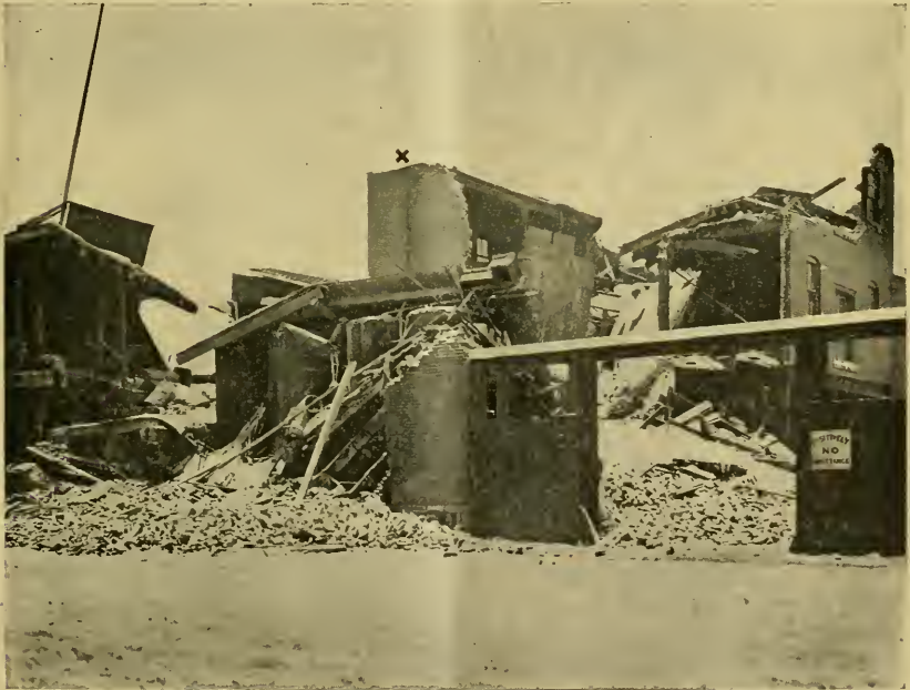
VIEW OF THE WRECKED PLANT.
