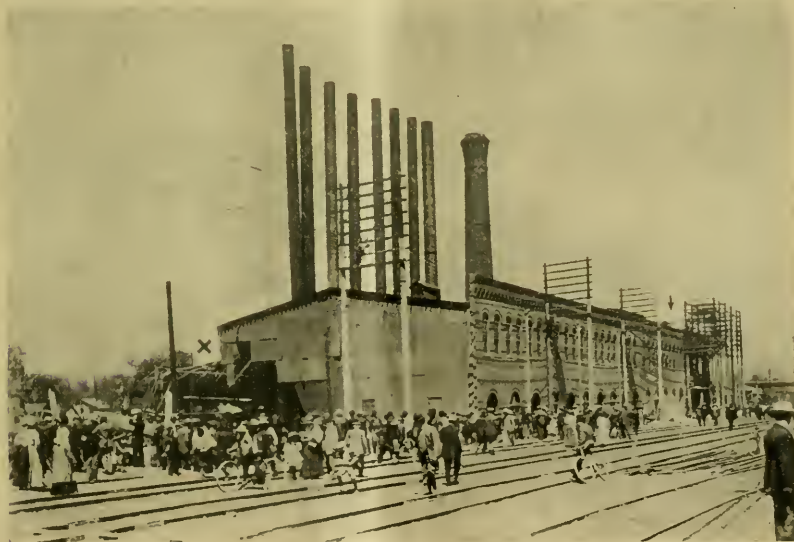
FIG. I.—GENERAL VIEW OF THE PLANT.
