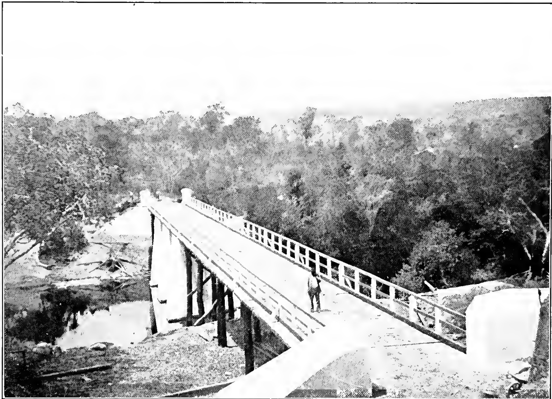
BRIDGE CROSSING RIO UNA, STATE OF BAHIA.
