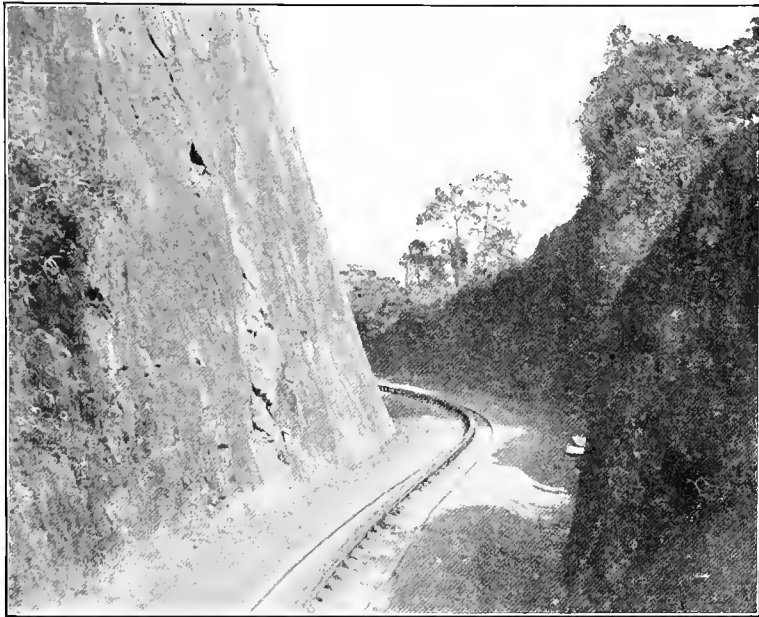
THREE-RAIL TRACK ON LEOPOLDINA RAILROAD, STATE OF RIO.
