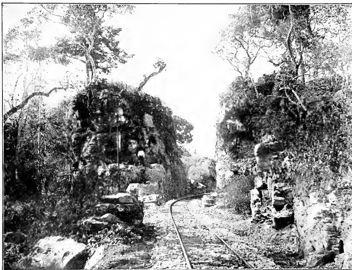
VIEW ON THE CENTRAL RAILWAY.
