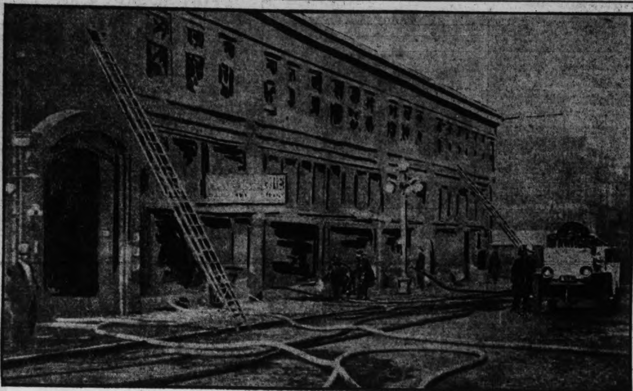
Firemen check blaze at fire wall line in centre of block.
