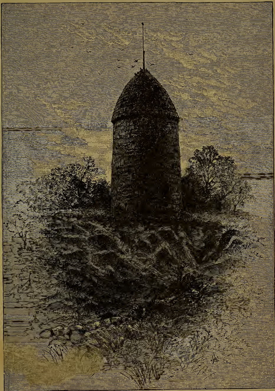
THE OLD POWDER-HOUSE AT SOMERVILLE.
