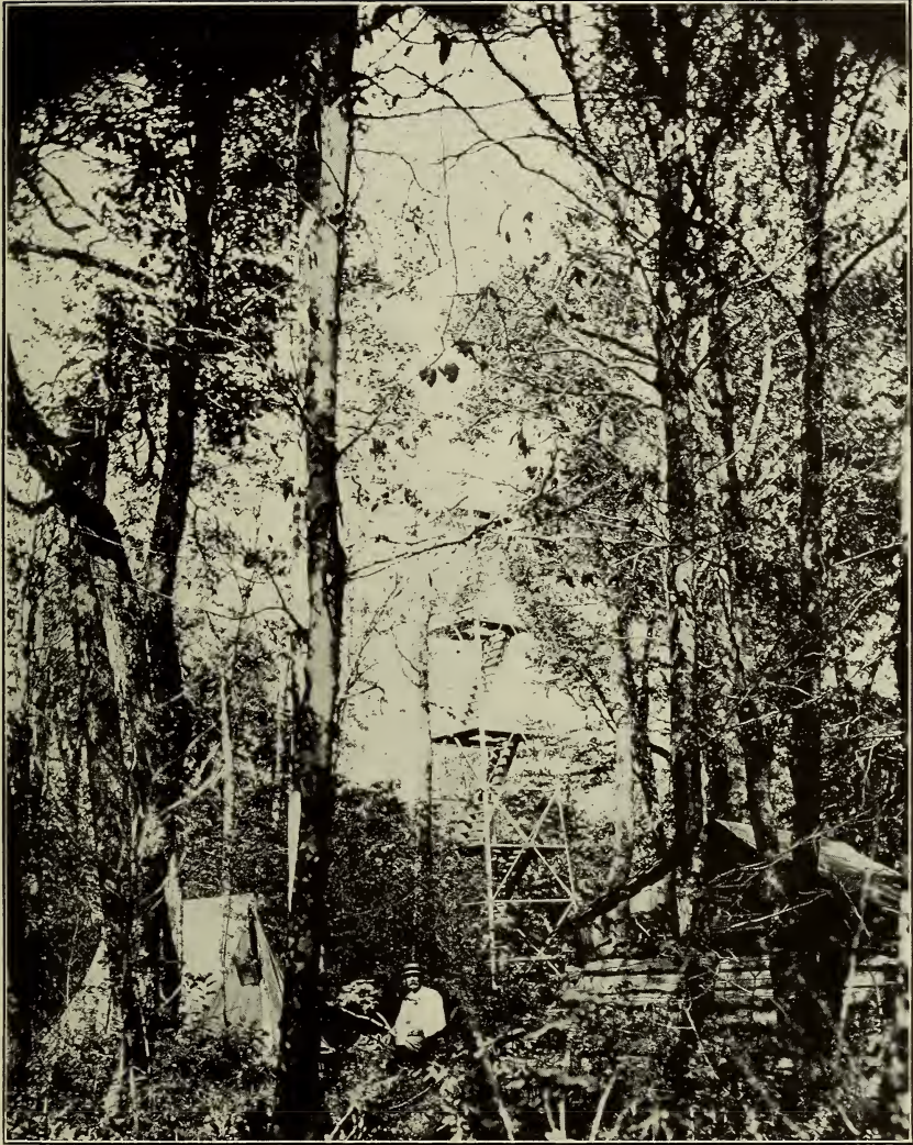
Steel Fire Lookout Tower on Belle Ayre Mountain (65 feet high), Pine Hill, N. Y.
