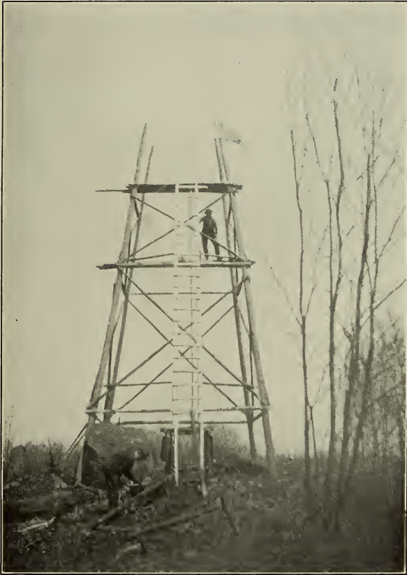
Observation Tower on Fort Noble Mountain, Herkimer County. Height 50 Feet.
