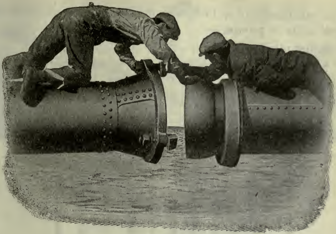
FIG. 1,674.—Parker pontoon pipe coupling being assembled.
