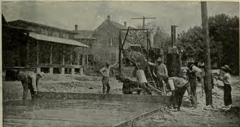
FIG. 1,709.—Standard street paving mixer at work.
