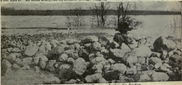
FIG. 1,672.—Spoil pile of rock from a 20 inch Bucyrus hydraulic dredge.
