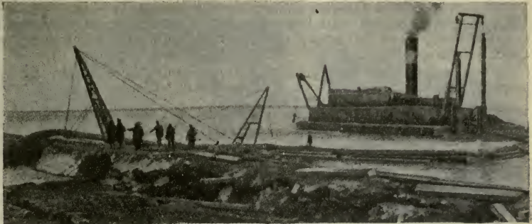
FIG. 1,670.—20 inch Bucyrus hydraulic dredge at work on the Great Lakes.
