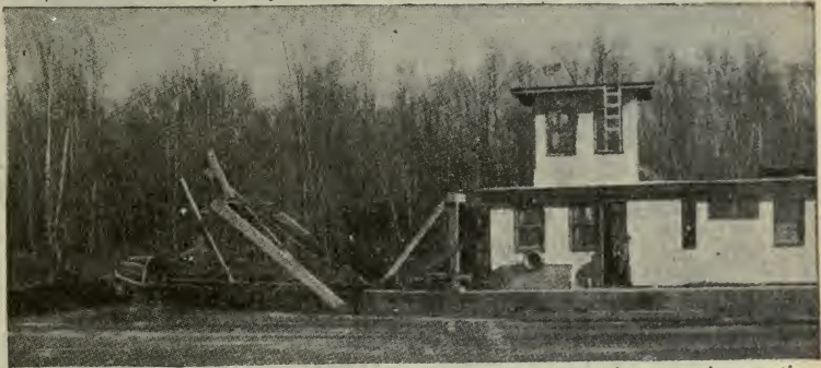
FIG. 1,671.—20 inch Bucyrus hydraulic dredge digging a canal, showing cutter in operation.
