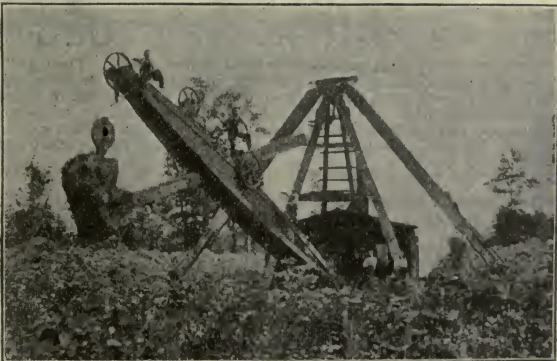
FIG. 1,659.—Marion dipper dredge cutting ditch through timbered country.
