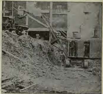
FIGS. 1,637 to 1,641.—Various types of Thew steam shovel. Fig. 1,637, type O shovel using horizontal crowding motion to excavate shallow sub-grade for paving; fig. 1,638, type O shovel with horizontal crowding motion excavating a through cut in road construction work; fig. 1,639, type O shovel using shipper shaft mechanism and long dipper stick in trench excavation; fig. 1,640 example of high lift work done by Thew shovel equipped with long dipper stick; lift is 20 ft. above level of wheels; fig. 1,641 example of how Thew shovel digs its way down to the level of the excavation.
