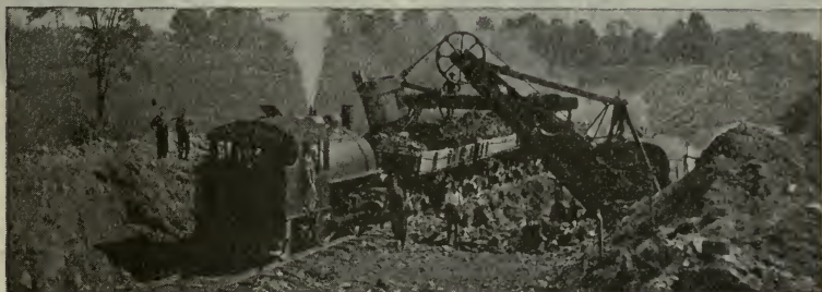
FIG. 1,644.—Bucyrus steam shovel in railroad work making a through cut.
