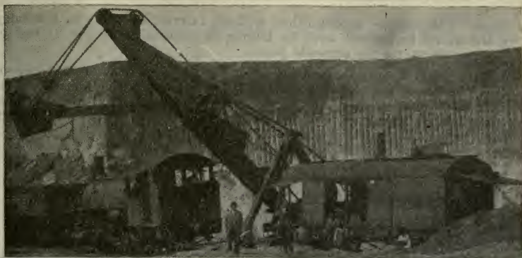
FIG. 1,643.—Bucyrus shovel with special long boom digging full height of 35 foot gravel and clay bank.
