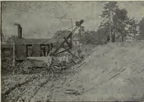
FIGS. 1,637 to 1,641.—Various types of Thew steam shovel. Fig. 1,637, type O shovel using horizontal crowding motion to excavate shallow sub-grade for paving; fig. 1,638, type O shovel with horizontal crowding motion excavating a through cut in road construction work; fig. 1,639, type O shovel using shipper shaft mechanism and long dipper stick in trench excavation; fig. 1,640 example of high lift work done by Thew shovel equipped with long dipper stick; lift is 20 ft. above level of wheels; fig. 1,641 example of how Thew shovel digs its way down to the level of the excavation.
