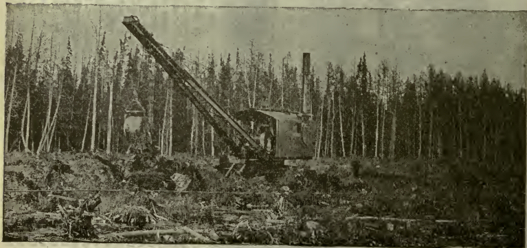
FIG. 1,652.—Bucyrus drag line excavator on caterpillar traction digging small drainage ditches.
