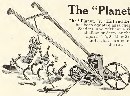
NO. 25 PLANET, JR., HILL AND DRILL SEEDER COMBINED WITH DOUBLE WHEEL HOE
