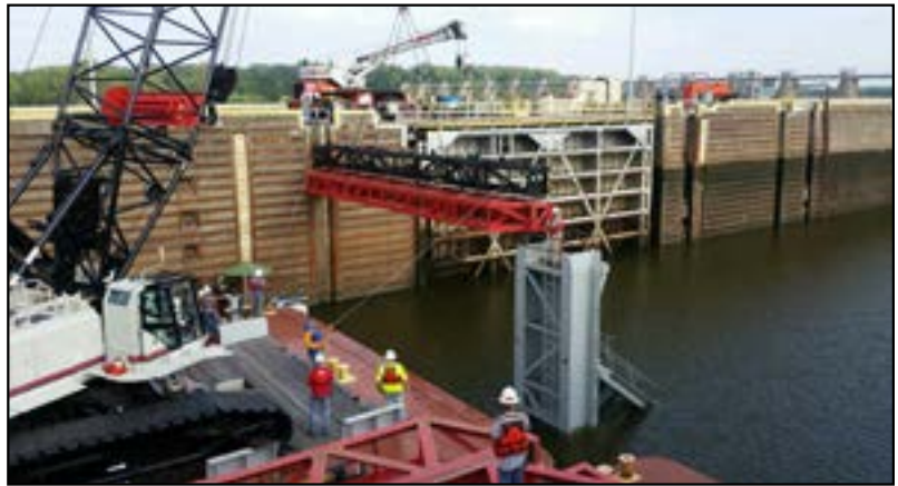
Lock 6 Setting Dewatering Bulkheads Figure 17 (see pg. 16) 2016: SWL District
