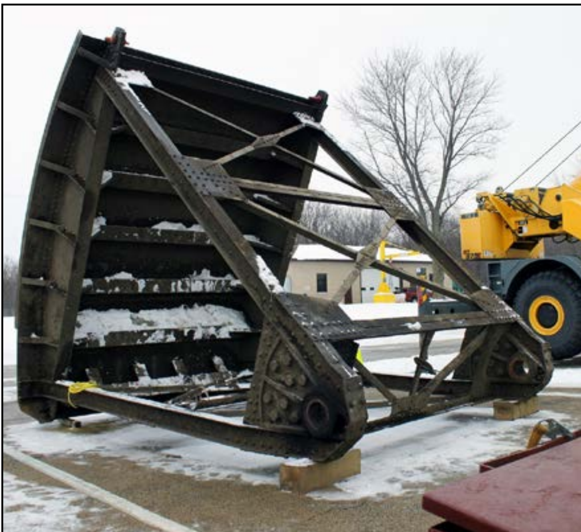
Lock 13 Tainter Valve removed for repairs, 2016 Figure 12 (see pg. 15) MVR District
