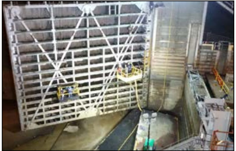
Lock Dewatering 2016: Lock 16 MKARNS Miter Gate Maintenance. SWT District
