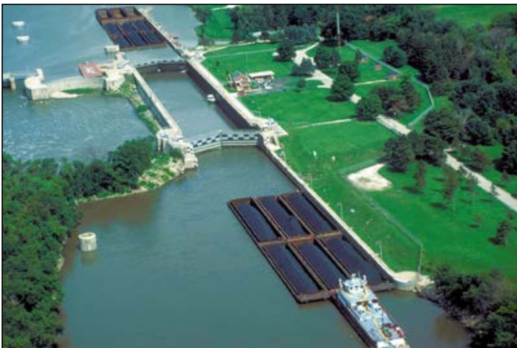
Dresden Island Lock - IWW Figure 16 600' chamber with 1200' tow broken into two cuts for lockages MVR District
