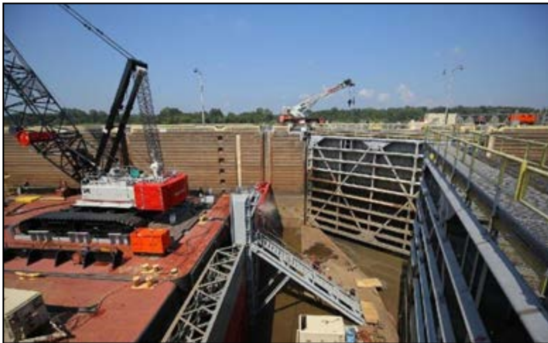
Lock dewatering 2016: Figure 15 (see pg. 16) Lock 16 MKARNS SWT District
