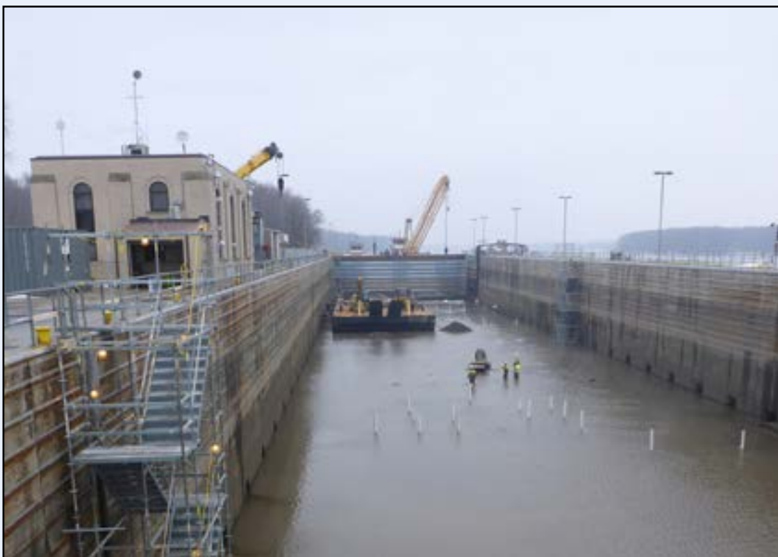
Lock dewatering 2016: Lock 13 Upper Mississippi River MVR District.
