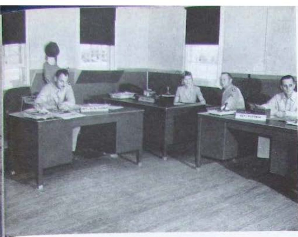
Post Signal Office.
