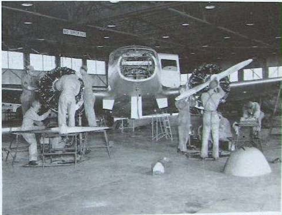
Installing Spark Plugs Propeller Inspection.
