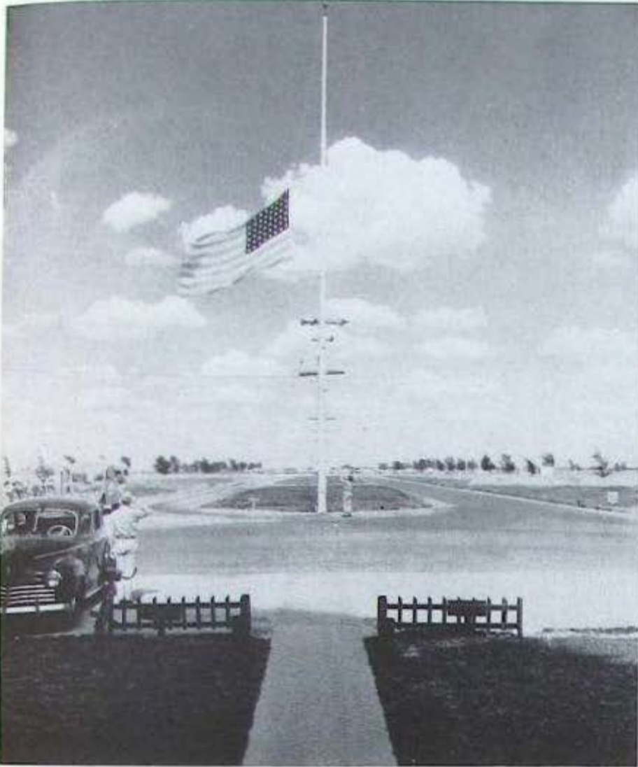
A View from the Headquarters Building Entrance.
