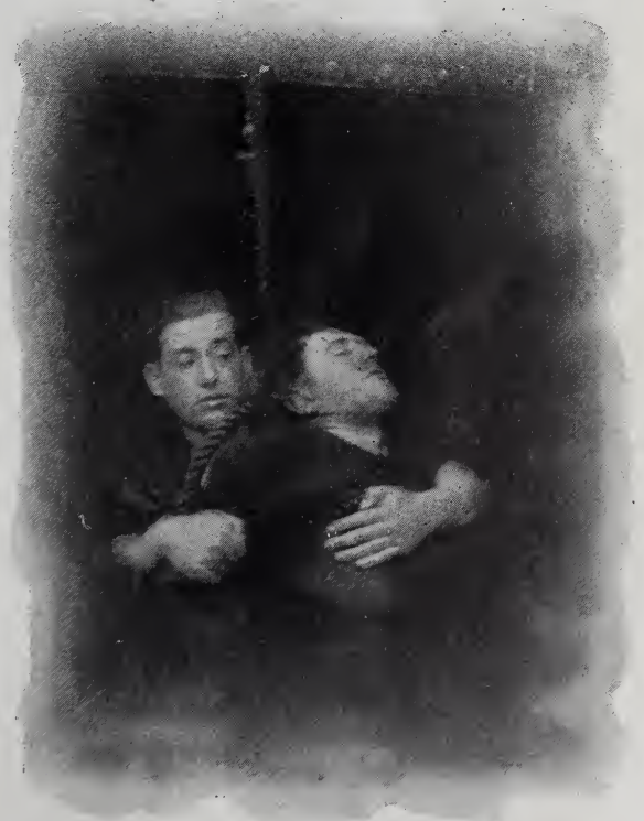
IN THE HEART OF THE CAISSON
